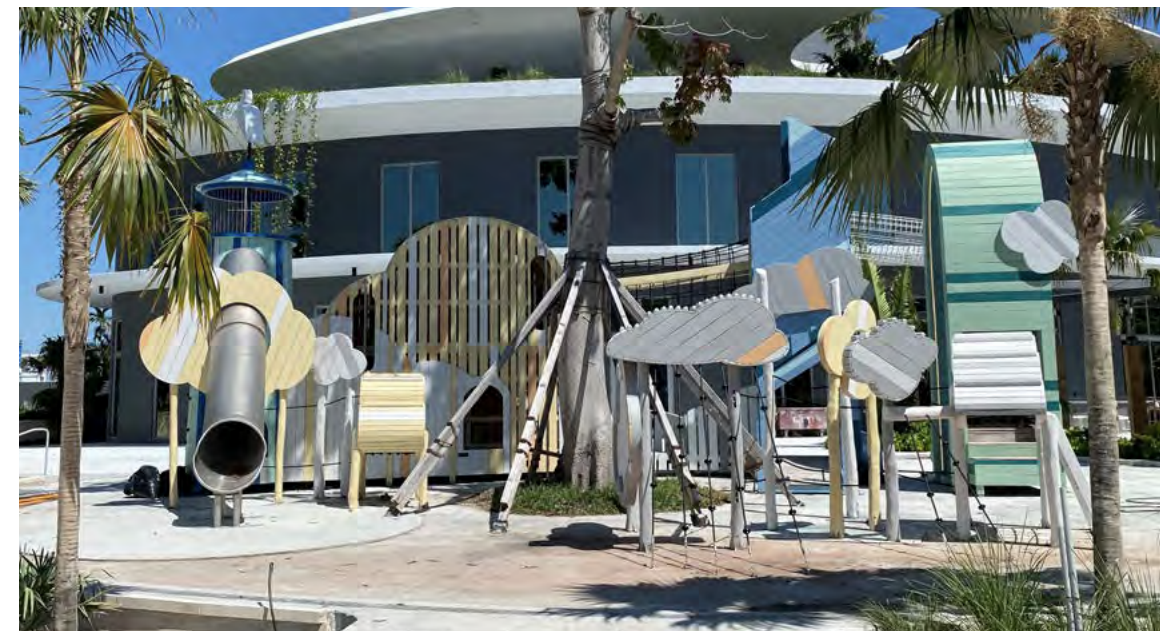
The under-construction playground at Waterfront Park, west of Bal Harbour Shops on Bal Bay Drive. Play components include multiple climbing towers (3-4), slides, and bridges.
