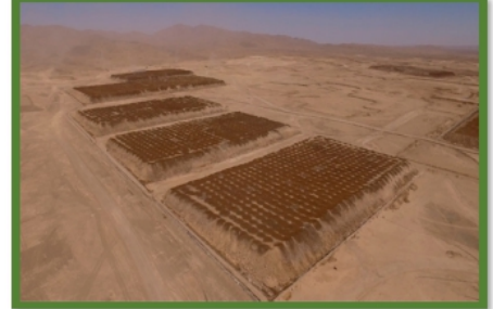
Figure 13-3. Pad Construction and Morphology in Nueva Victoria Mine (caliches)
