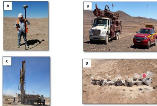
Figure 8-1. A) Drilling Point Marking B) Drill Rig Positioning C) RC Drilling D) RC Samples at Platform
