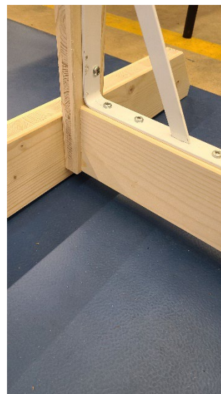
Iron bracket for reinforcement
