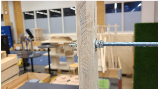
Threaded rod mounting inside
