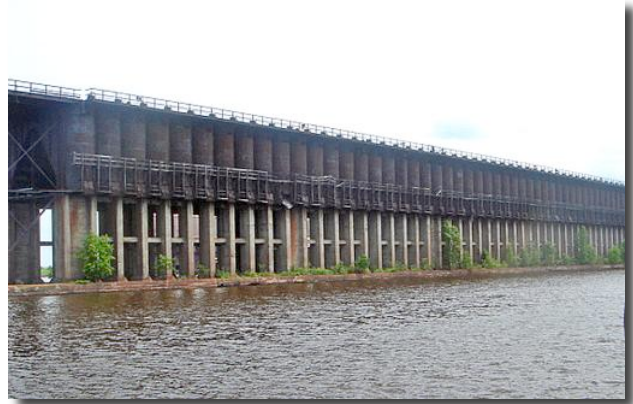
Above: The abandoned ore dock Photo credit: Dave Evans
