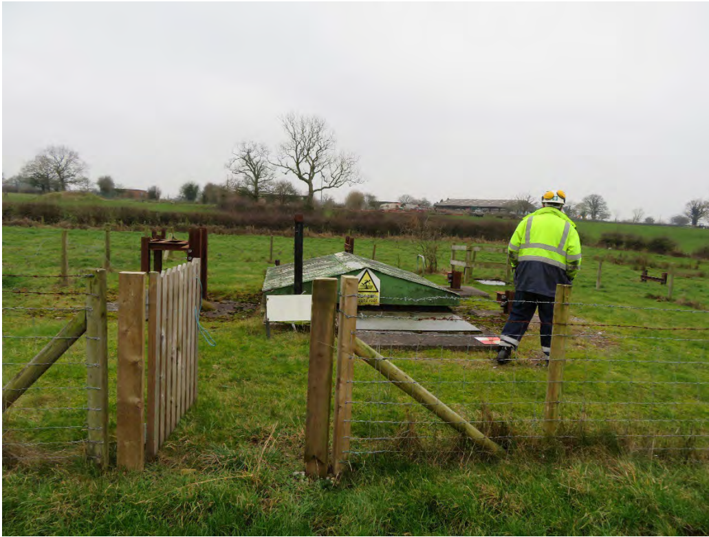
Cavern T11. Entrance
