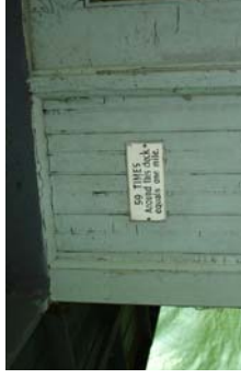
Exterior details such as this sign should be preserved
