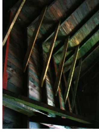
Current roof rafters and support
