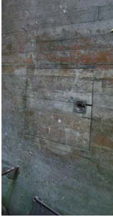
Floor storage space
