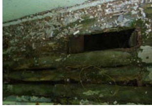
Damaged wood on lower deck
