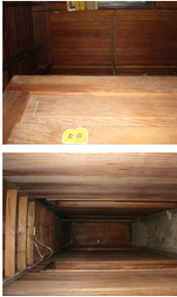
Most interior woodwork remains in good condition
