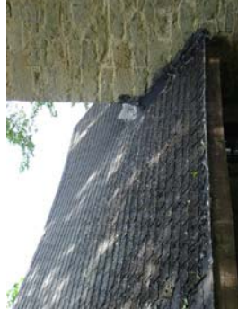
Current roof condition
