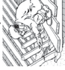
Loose fill insulation
