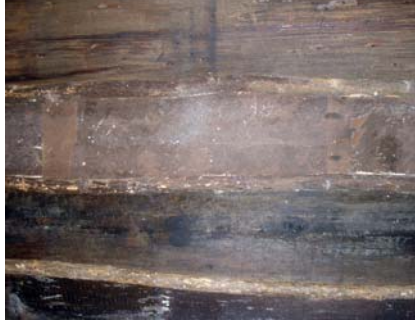
Original interior wood paneling
