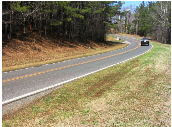
Secondary road in the Haw River subwatershed
