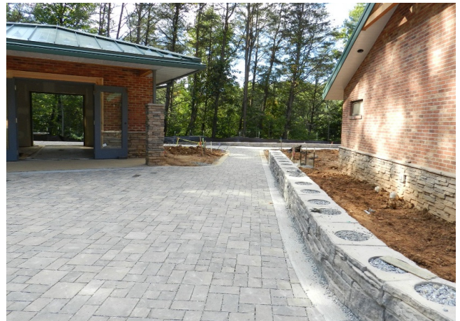
Permeable pavers installed at a rest area
