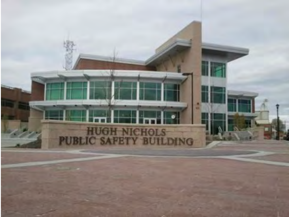
FIGURE 13. NAMPA POLICE DEPARTMENT BUILDING
