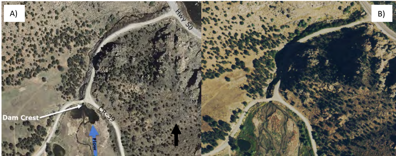
Figure 4: Harry Walker Dam A) aerial image taken in 2016 pre-fire/flood showing capacity, and B) post-fire/flood showing sedimentation and braided channels overtopping the dam crest.
