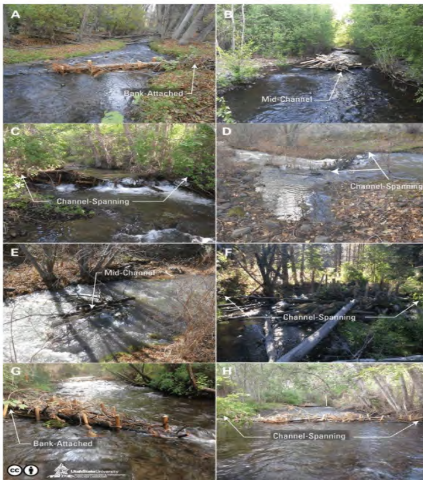
Figure 5: Images of PBR treatments that show Channel-Spanning BDAs and PALS, bank-attached PALS, and mid-channel PALS.
