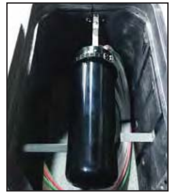
90° Splice closure mounting
