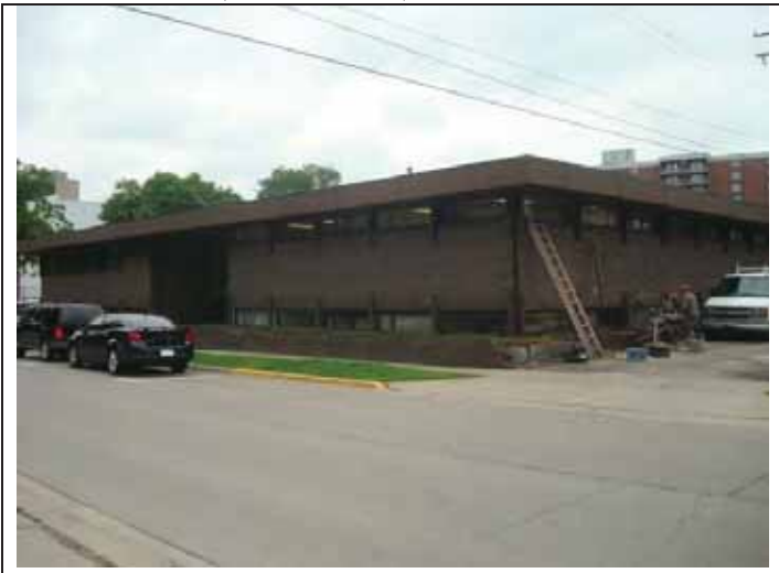
23. View of the south adjoining office building located across an alley (751 Chestnut Street)
