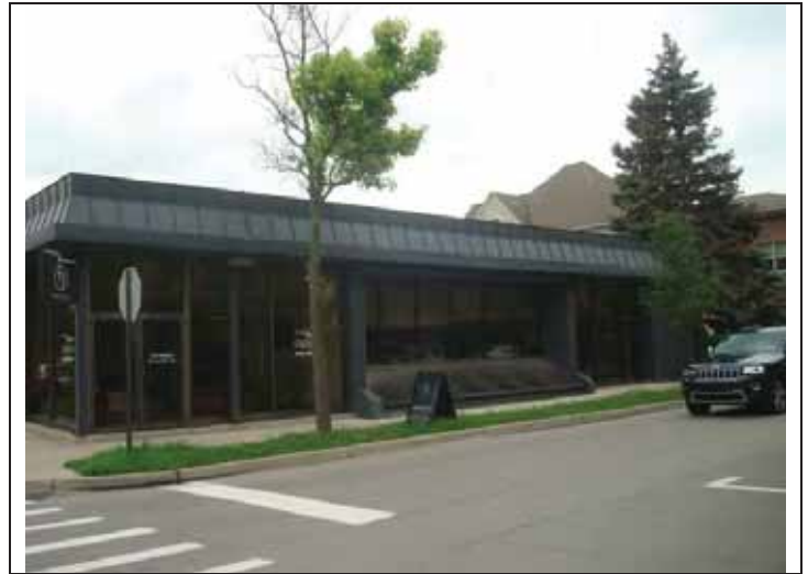
2. View of the north elevation of the building
