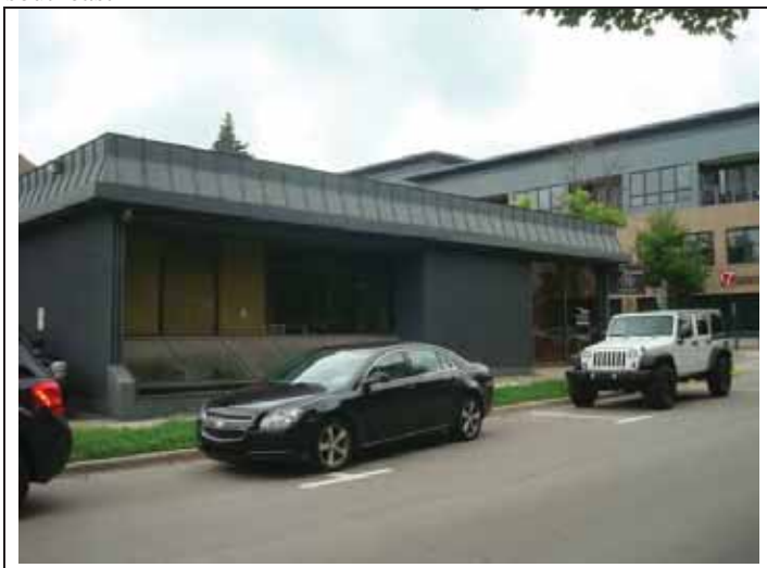
3. View of the east elevation of the building
