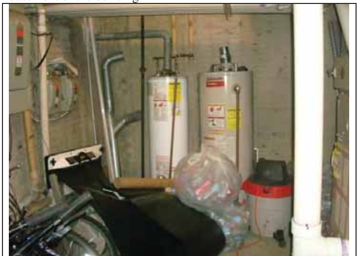
12. View of the furnace room in the basement of the building
