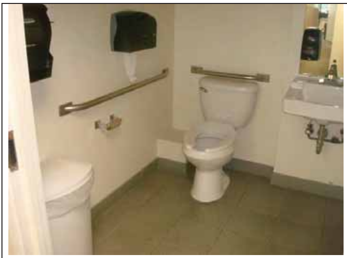
7. View of a restroom in The Student Connection tenant suite located on the first floor of the building (770 Forest Avenue)
