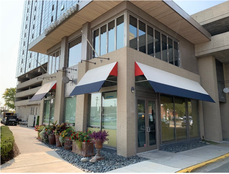
Existing Awnings – SW Corner
