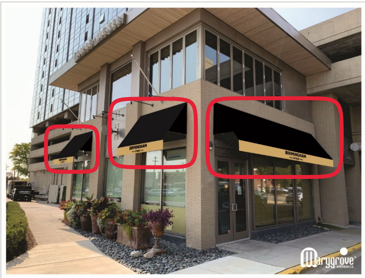
Existing Awnings – SW Corner
