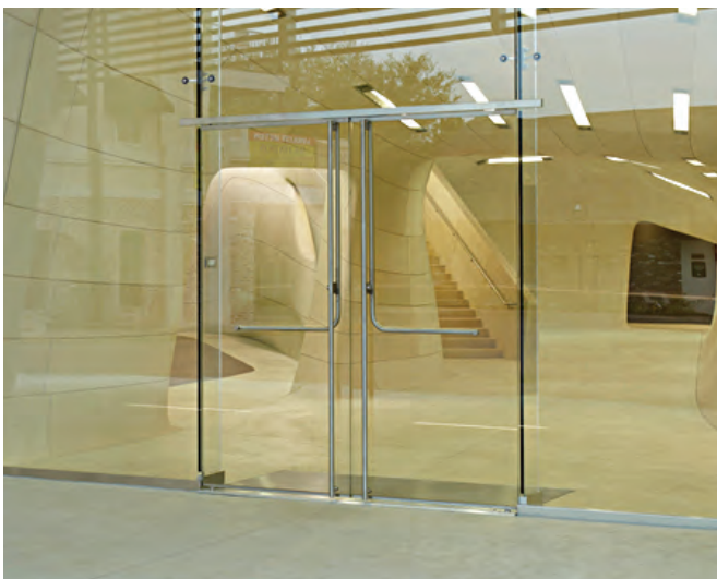
FRAMELESS GLASS DOORS & BUTT GLAZED WINDOWS AT REAR WINTERGARDEN WALL
