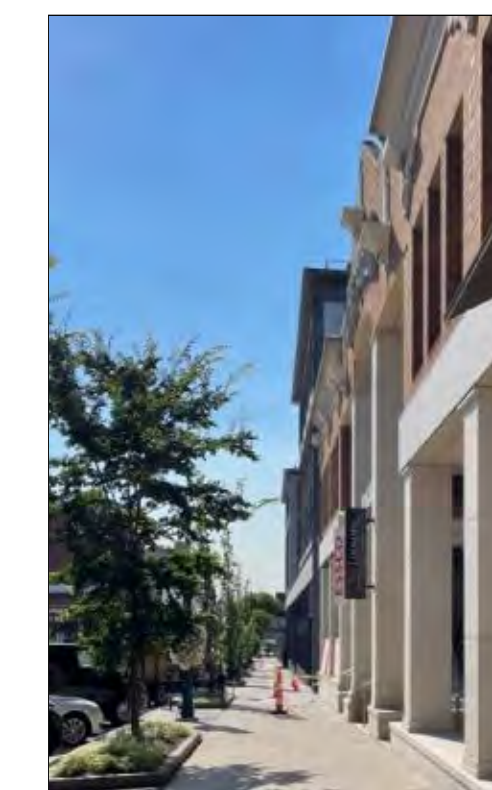
E.1 EXISTING EXTERIOR Old Woodward / Merrill Street Plaza Bldg - Looking South
