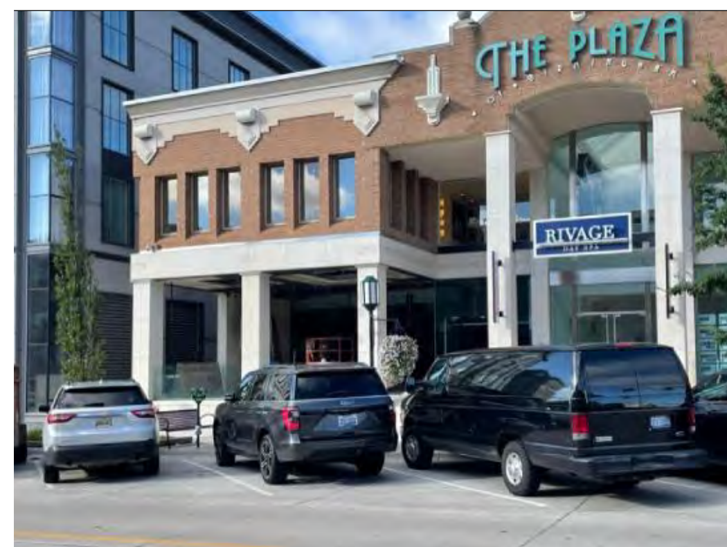
A EXISTING EXTERIOR South Portion of Plaza Bldg - Looking West
