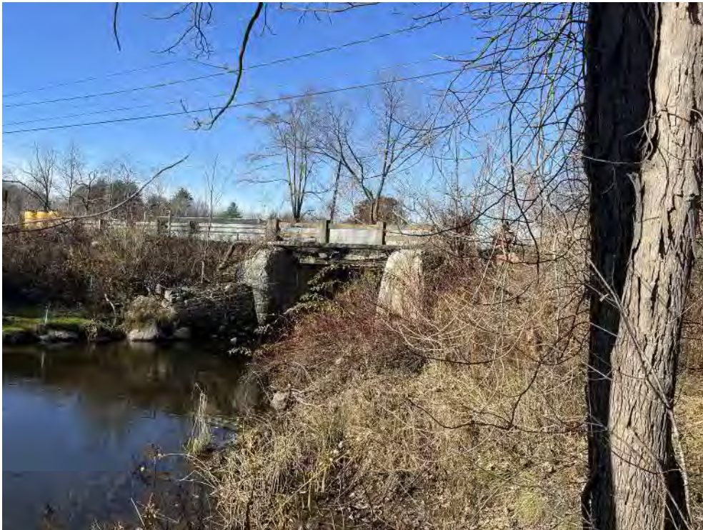
View of the southern side of the Rosemont Street Bridge—facing northwest.
