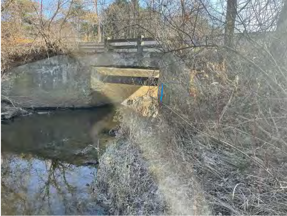
View of the northern side of the Rosemont Street Bridge—facing southeast.
