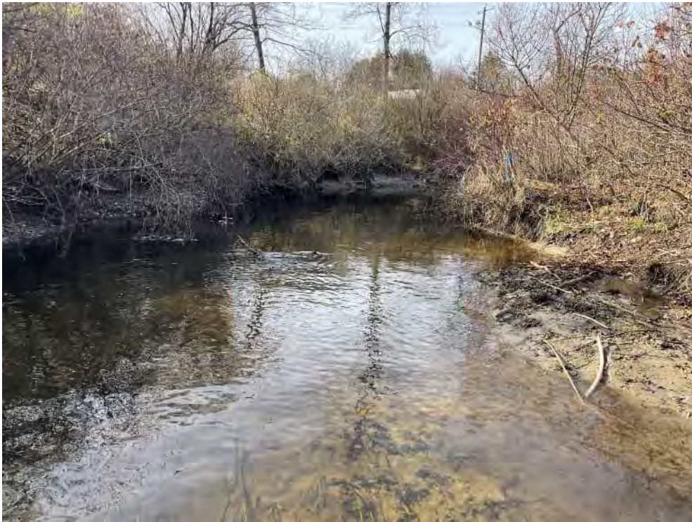
View of the B2-100 Series Bank north of the Rosemont Street Bridge—facing northwest.
