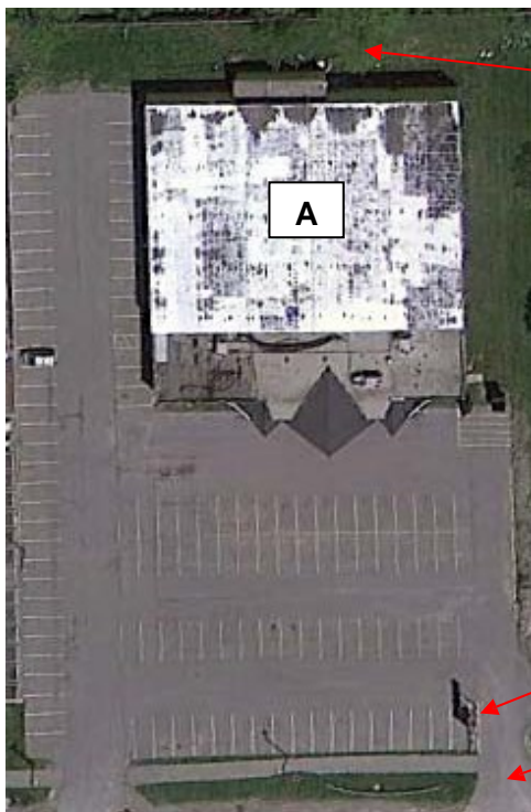
Existing Site Conditions
