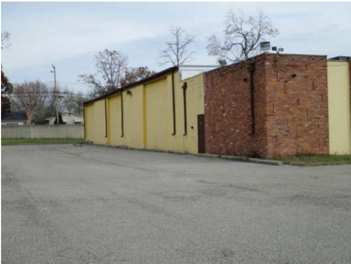
North Side of the Building
