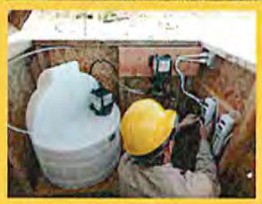
Technician installing the reservoir, pump and timing system
