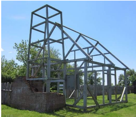
“Ghost frame” structures, created in other parts of the state and country, provide inspiration for how the Briggs House could be reflected in the new design.
