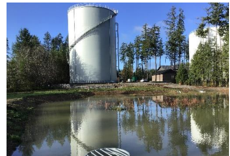
Second reservoir added to support maintenance and redundancy, existing detention storm pond modified to handle additional impervious surface at Hawks Prairie Reservoir
