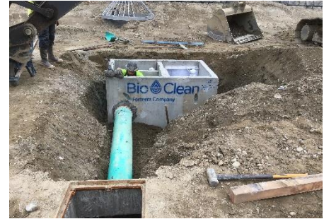
New stormwater system tying into a new filter vault to treat the added impervious surface associated with the Hawks Prairie Reservoir “Sister Standpipe” project
