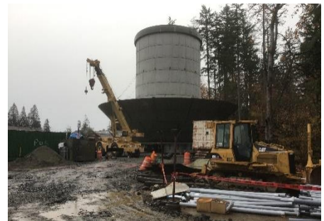
Constructing the Terry Cargil Reservoir
