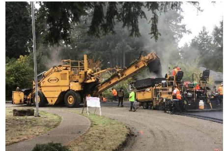
Laying asphalt in the Carpenter Hills neighborhood in 2023
