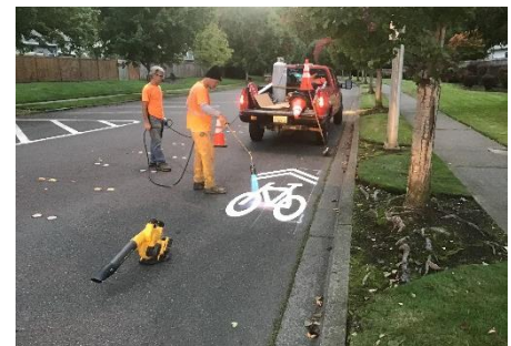
Applying shared lane thermoplastic bicycle symbols
