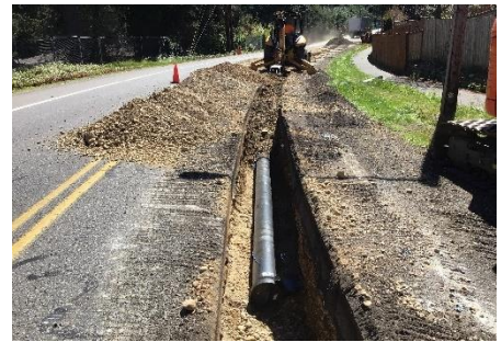
Installing a new water main and valves/appurtenances as part of the water replacement utility improvements at Carpenter Rd
