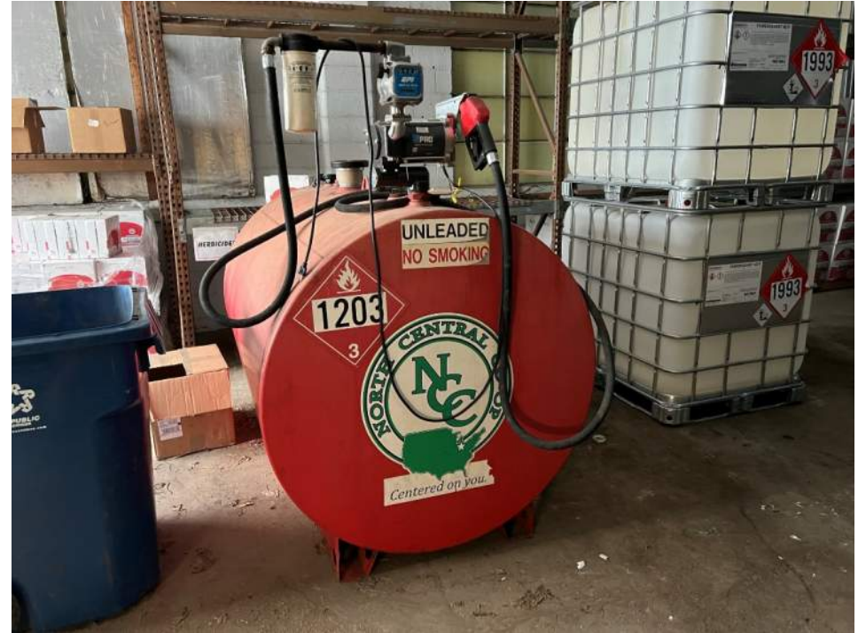
Chemical and fluid storage in Building B
