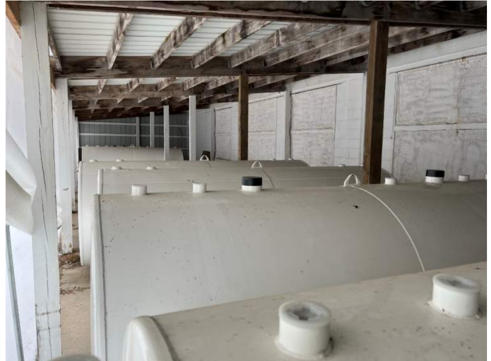
Empty AST storage in Building B
