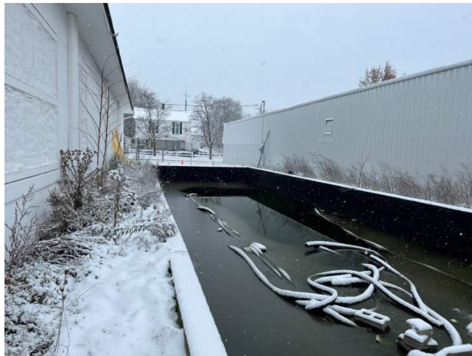
Dike containment system between Buildings B and C
