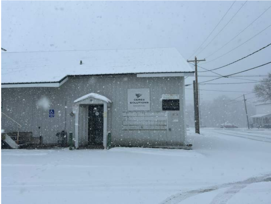
East side of Building A
