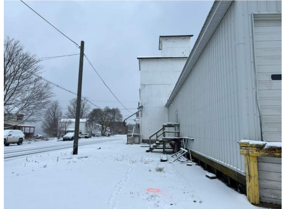
West side of Building A
