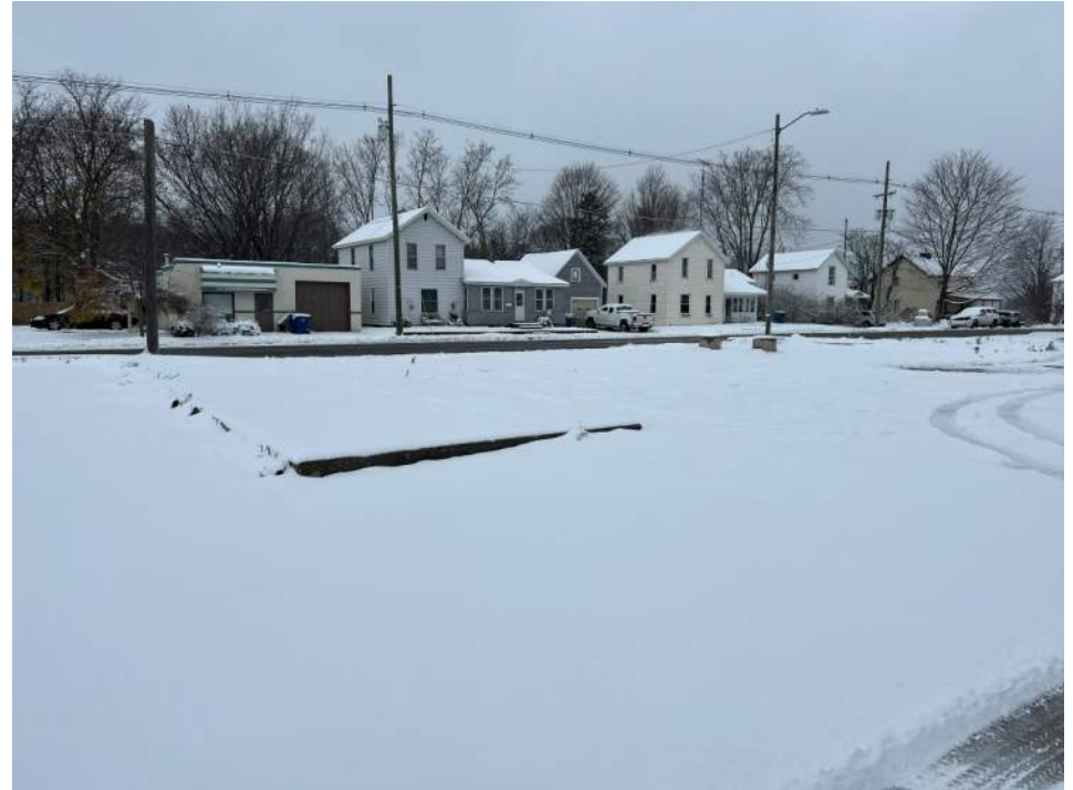
Foundation of former building west of Building D
