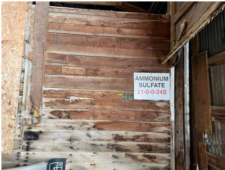
Former fertilizer storage in Building D
