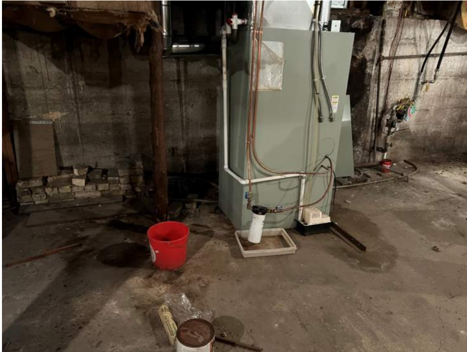
Basement of Building A
