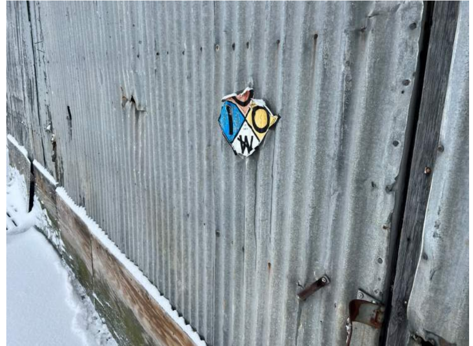
West side of Building D
