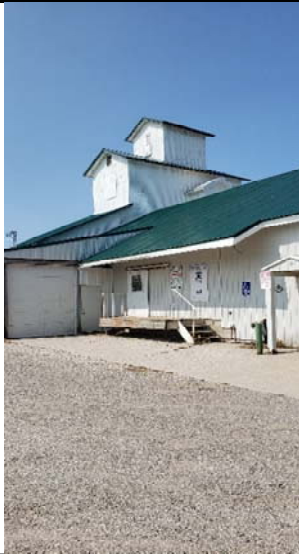
Subject Property - Grain Elevator
