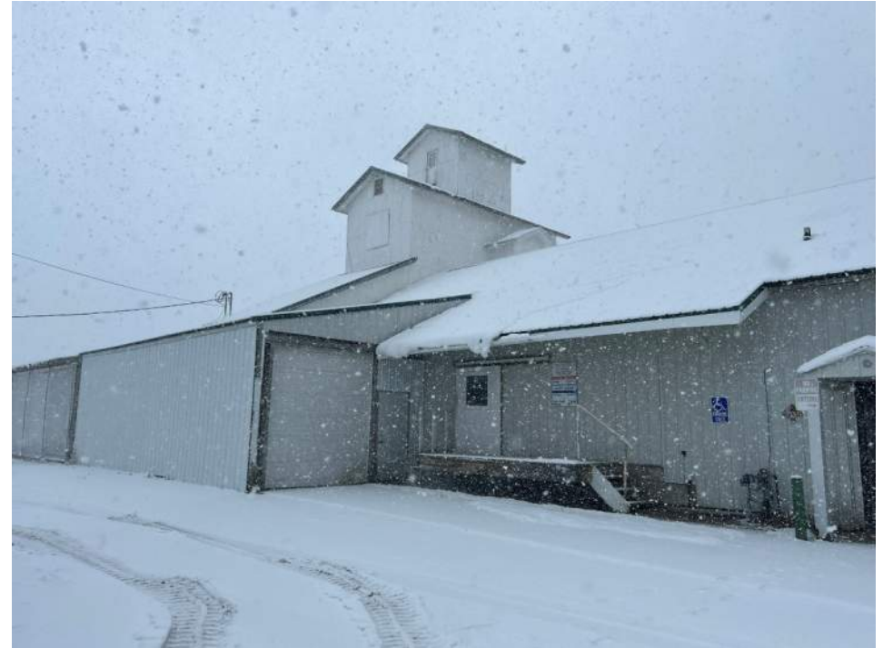
East side of Building A
