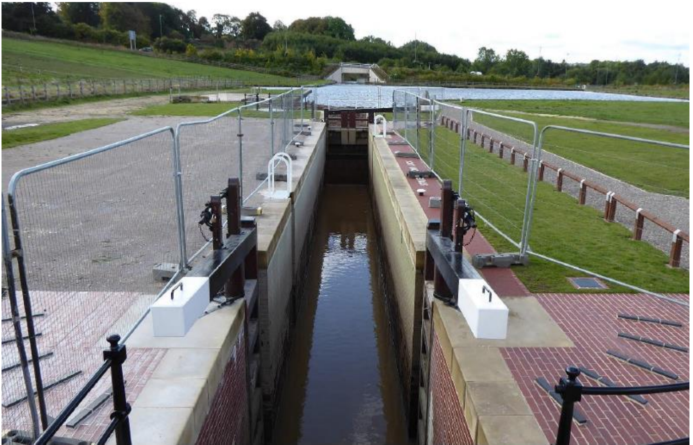
New Lock at Staveley Town Basin
