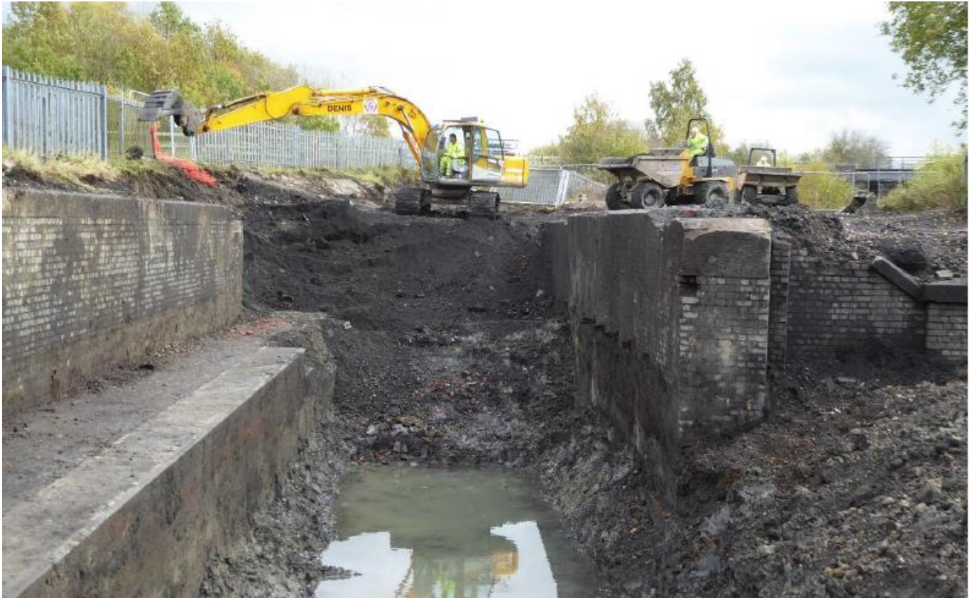
Uncovering of railway bridge under DCC Licence
