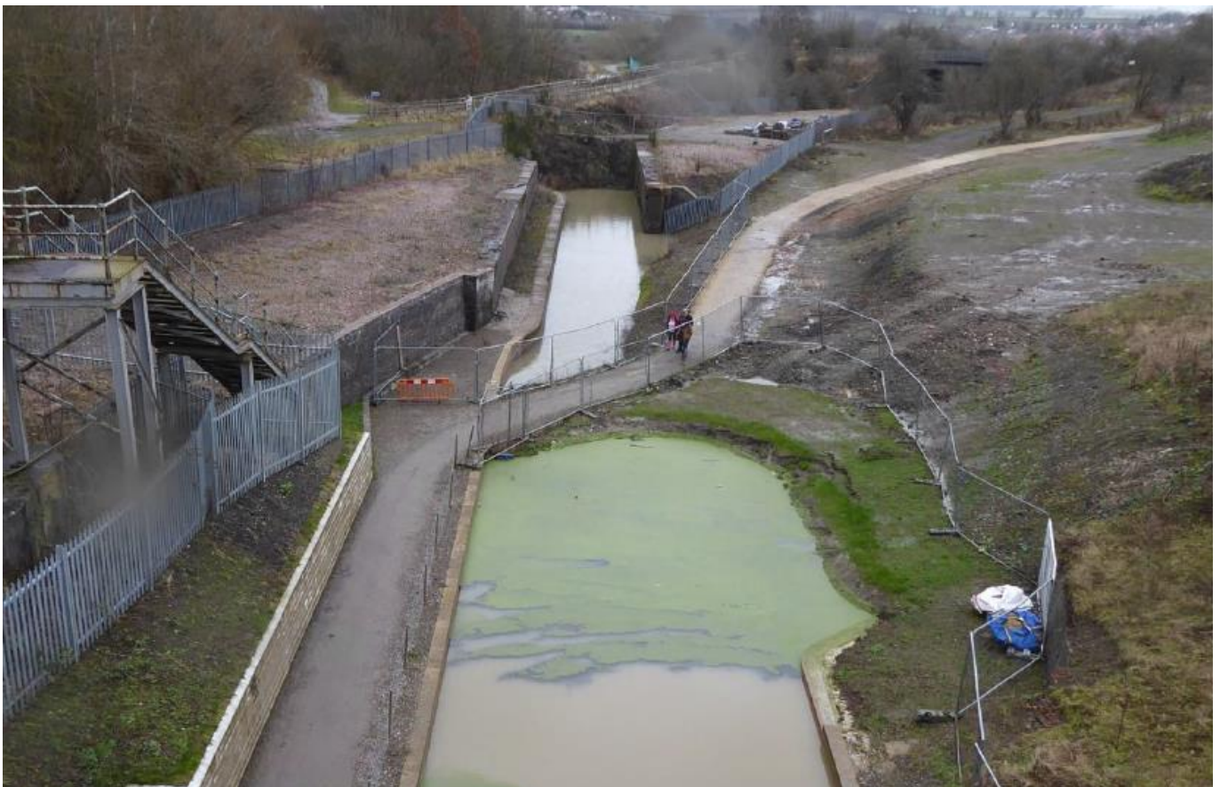
Looking east from Eckington Road bridge
