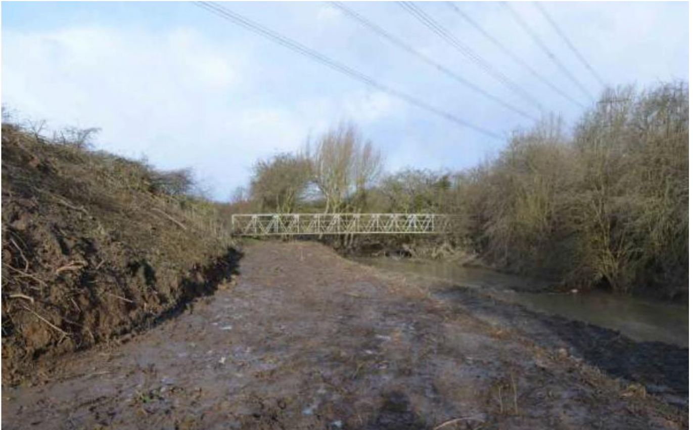
Existing Doe Lea bridge crossing
