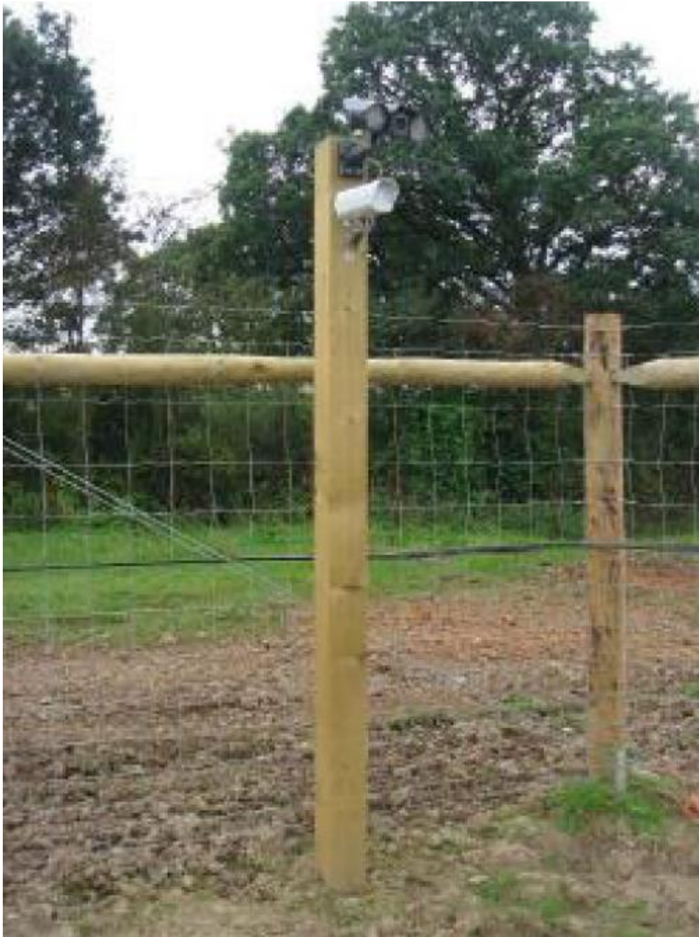
Typical CCTV camera and pole
