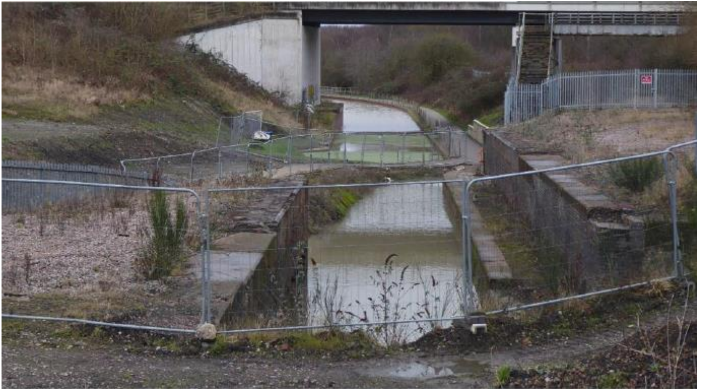
Looking towards Eckington Road bridge from east
