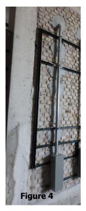
**Vertical Installation** – (Figure 4) – Vertical runs require an enclosure (pull box) be installed at the bottom of the raceway. The bottom raceway must exit through either the back or side wall of the enclosure. Vertical runs may utilize an enclosure (pull box) elsewhere within the system. The cable(s) shall enter and exit through the top and bottom of the enclosure.
