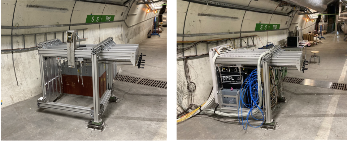
Figure 14: Mechanical support of the target system after the installation (left) and fully loaded with wall boxes and SciFi planes (right).
