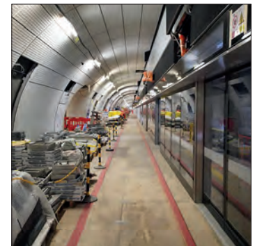
Crossrail: hugely complex
