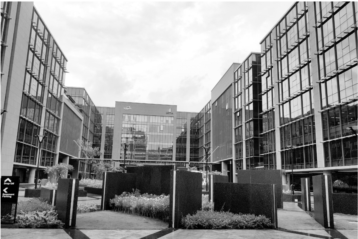
Sattva Knowledge Court Commercial Building for M/s Darshita Hi-Rise Pvt Ltd at Bengaluru, Karnataka.
