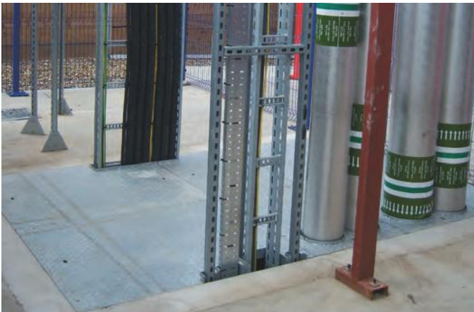
PS2100 Special Multiple cover and frame, this cover was installed at the Royal Mail Sorting Office in Croydon. This cover required multiple cut outs to allow for various sized pipework and cabling to pass through into the chamber below.
