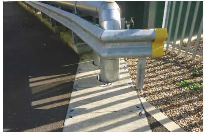
PS4600 FACTA D Continuous duct run concrete infill installed at GlaxoSmithKline. This is just one section which contained 4 specially designed trays to accommodate 2 pipes to pass through into the chamber. The length of this duct run was over 30m.
