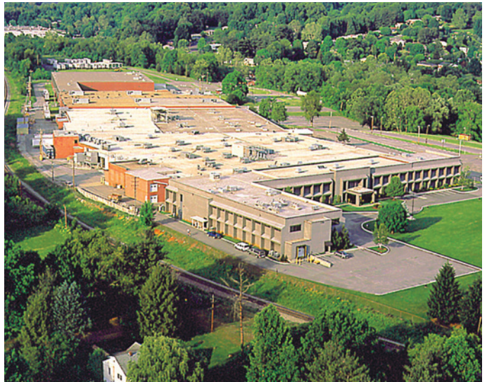
AERUS MANUFACTURING PLANT | BRISTOL, VA
