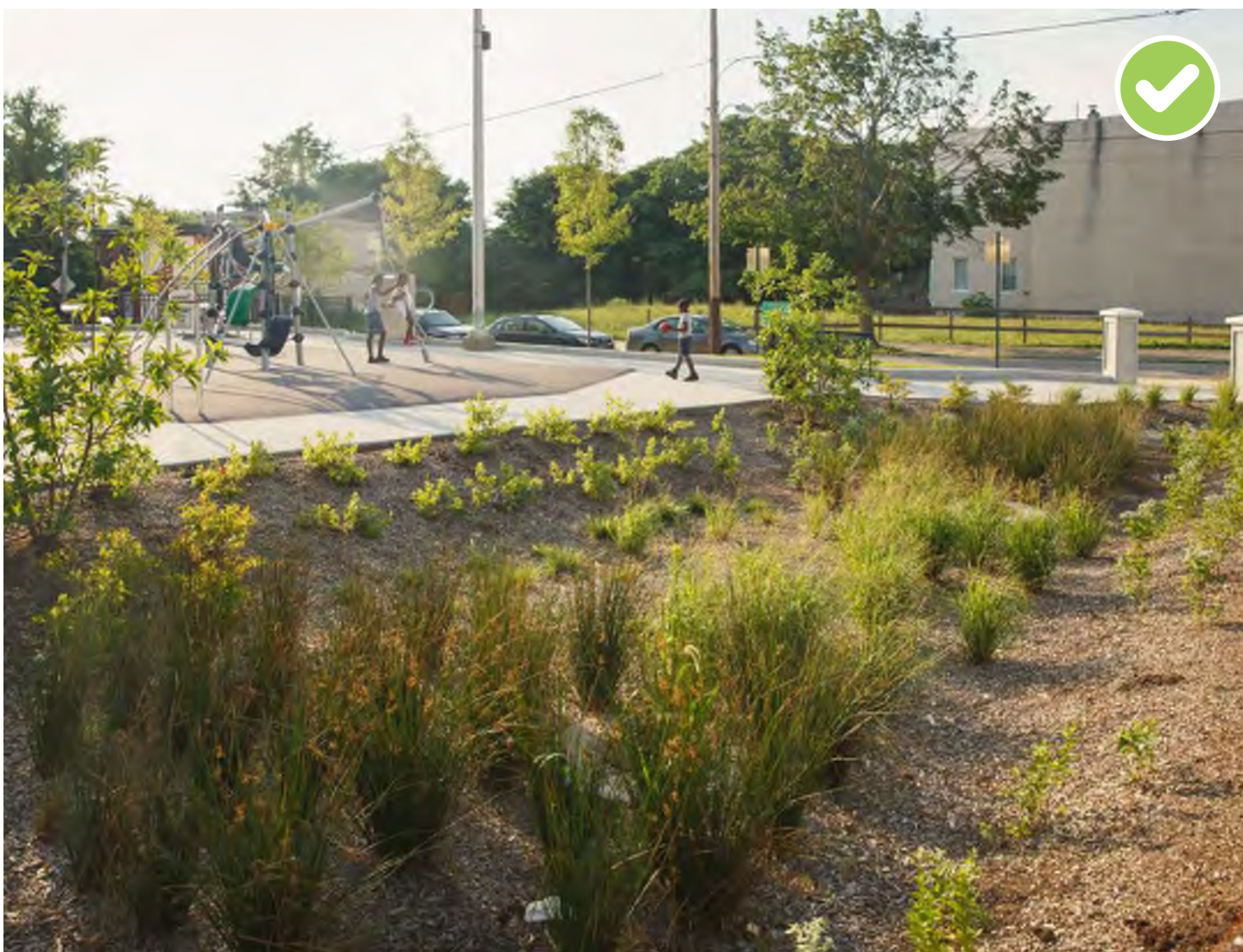
This newly planted rain garden built in at a playground manages runoff from the site and surrounding roadways.
