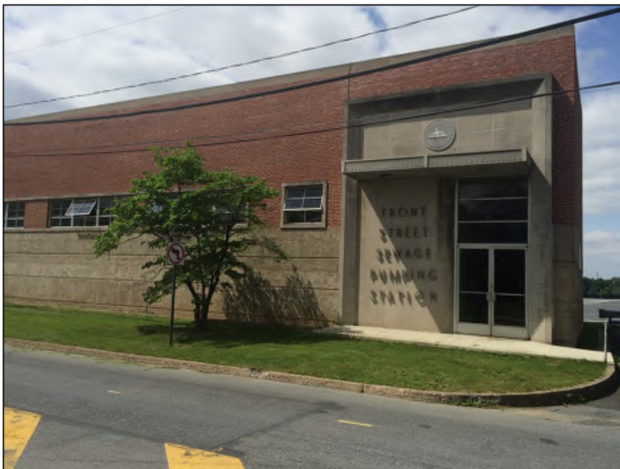
Figure 4.3-1 Front Street Pump Station
