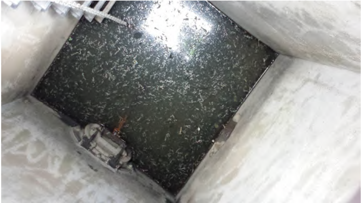
Flood Chamber with Flood Gate shown
