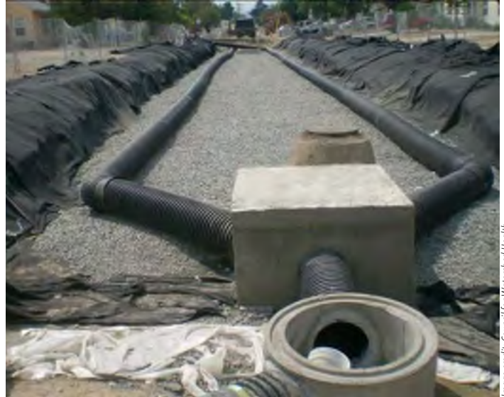
A storage/infiltration trench during construction, prior to backfill.
