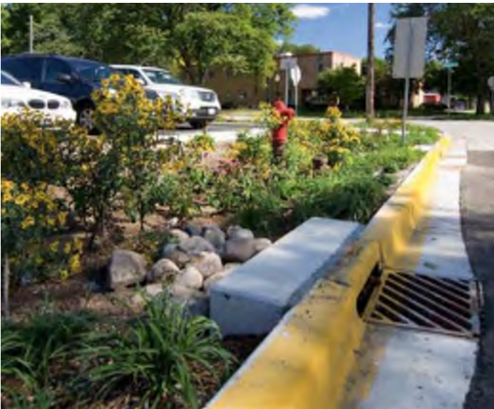
A rain garden designed to take stormwater runoff from the road through the use of a green inlet and splash pad.
