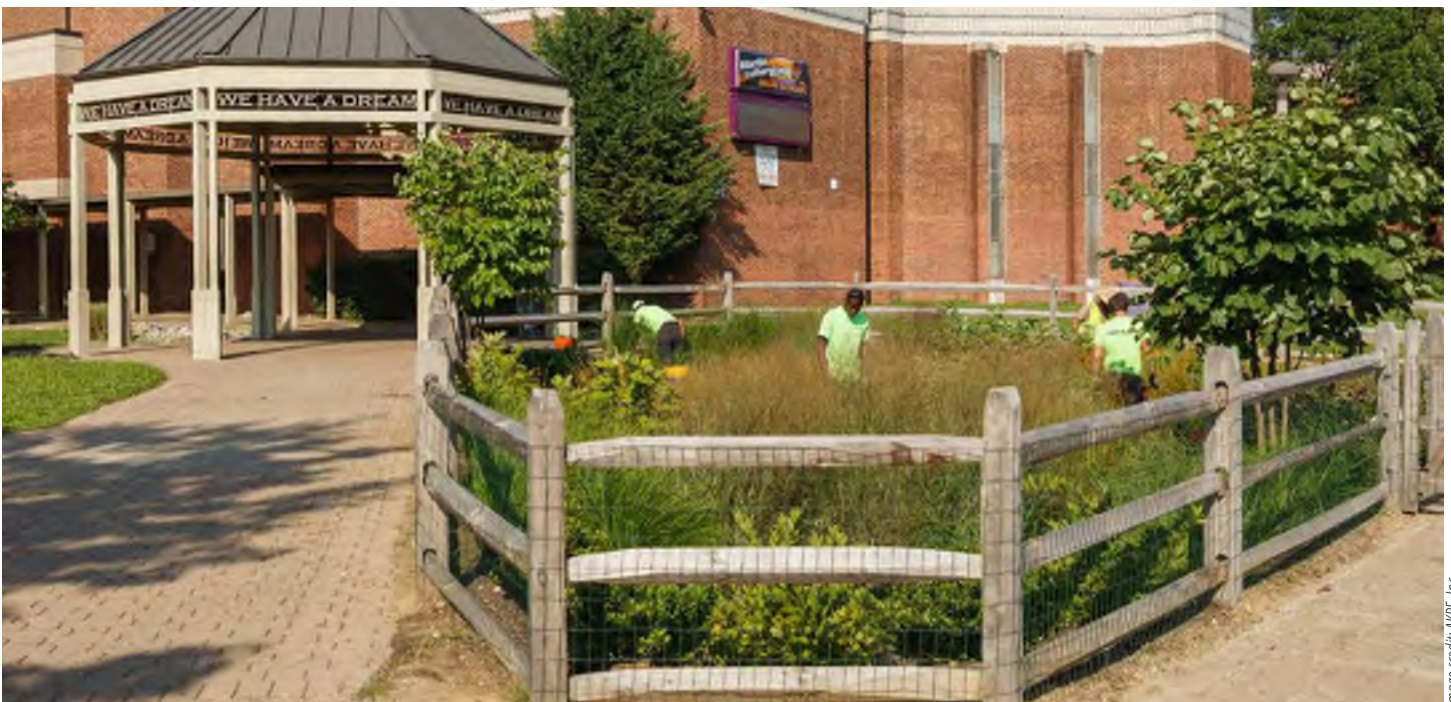
A field crew performing surface inspection and maintenance in a rain garden.
