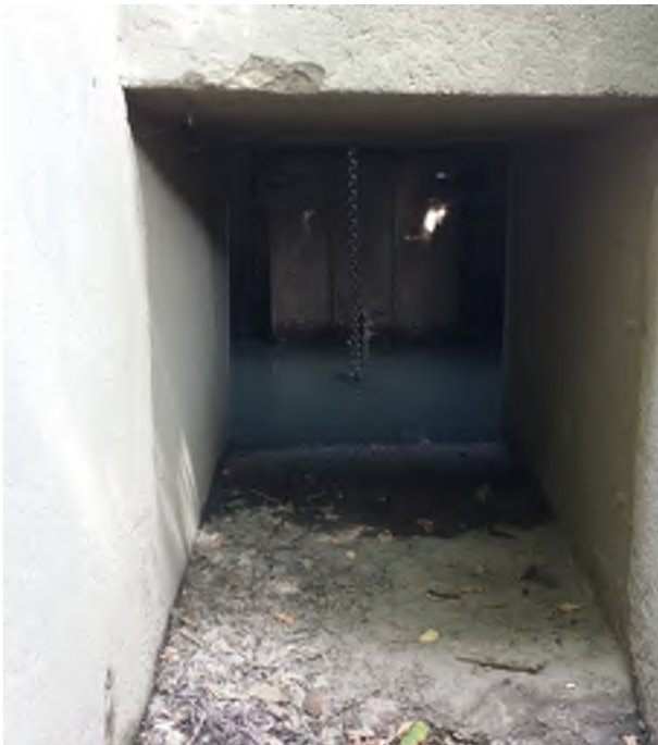
Figure 4.2-2 Photographs of Typical CRW CSO Outfalls and Flap Gates
