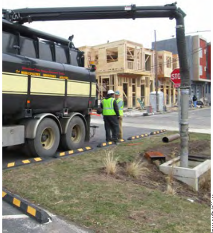
Maintenance crew using a jet-vac to clean rain garden pipes.
