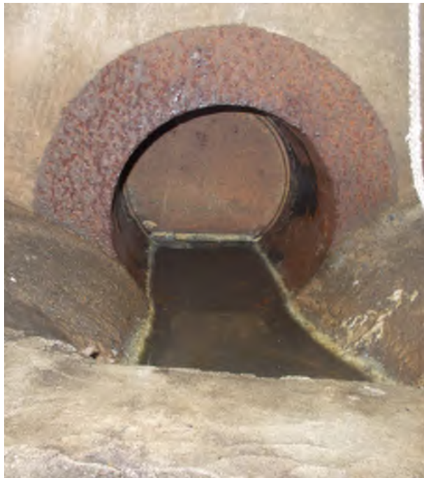
Figure 4.2-2 Photographs of Typical CRW CSO Outfalls and Flap Gates
