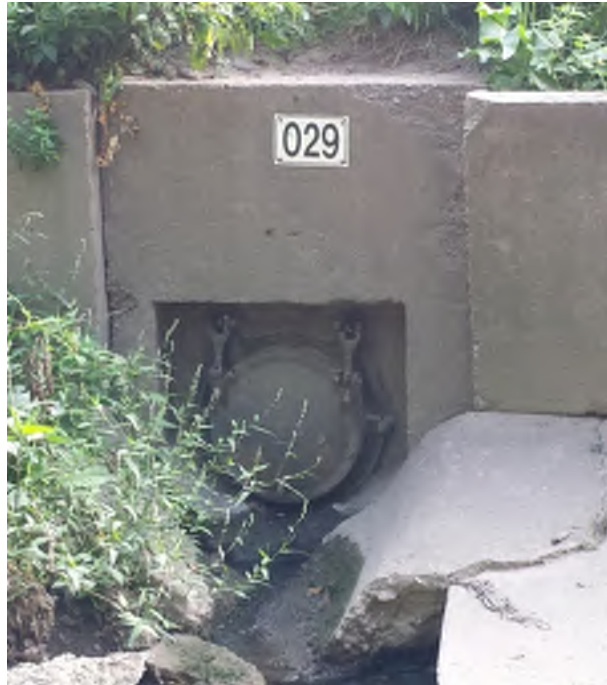
Flap Gate (viewed from diversion chamber)
