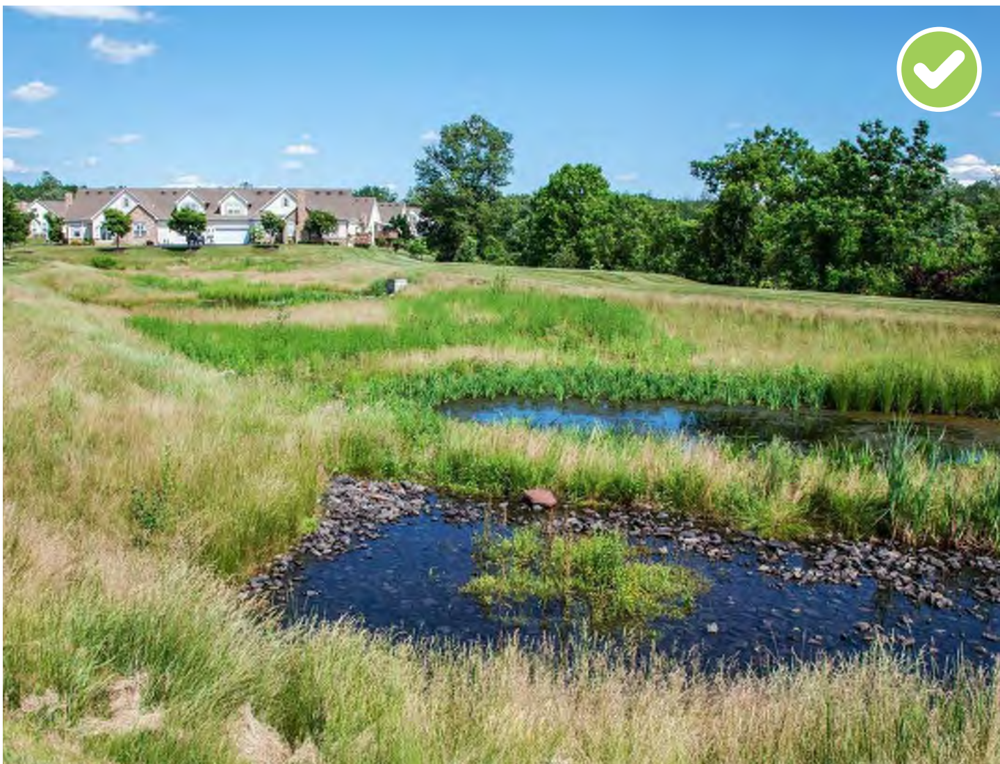
A stormwater basin planted with native trees, shrubs, and perennials throughout the entire extents can mimic a naturally occurring pond.
