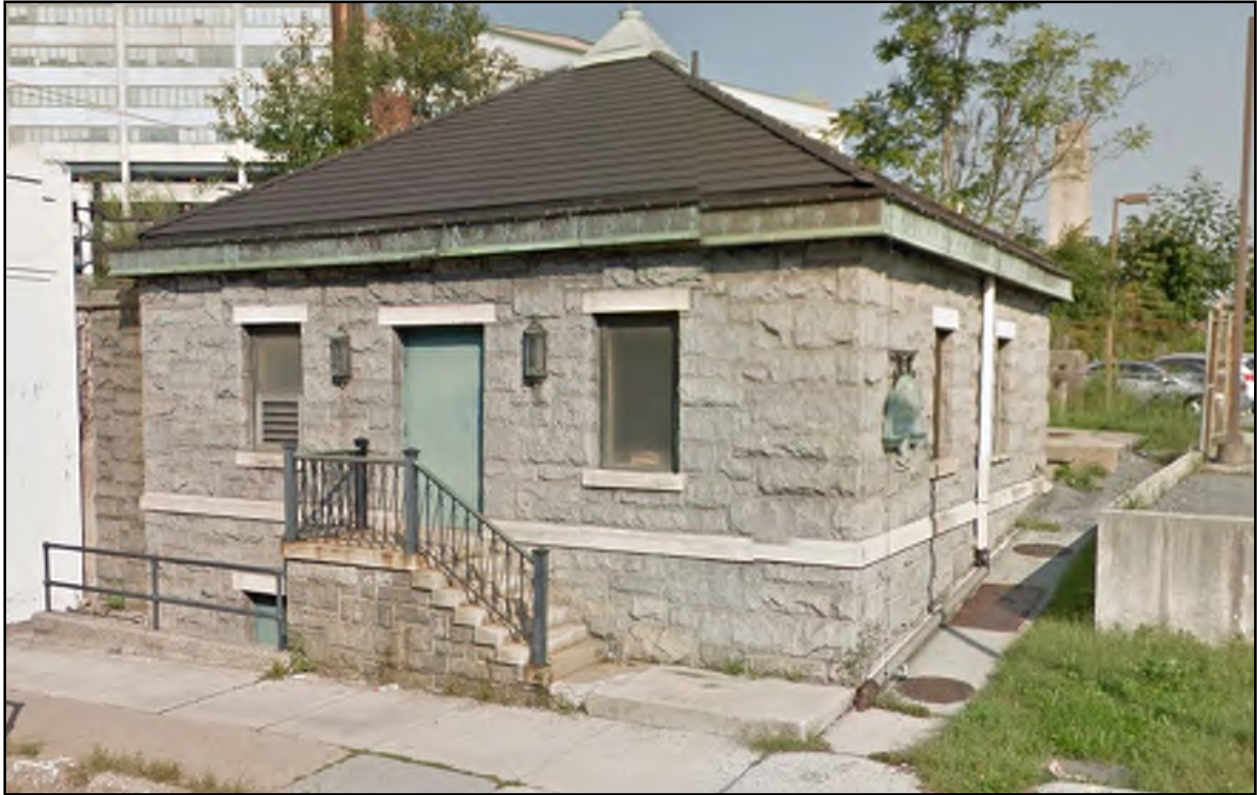
Figure 4.3-13. Market Street Pump Station
