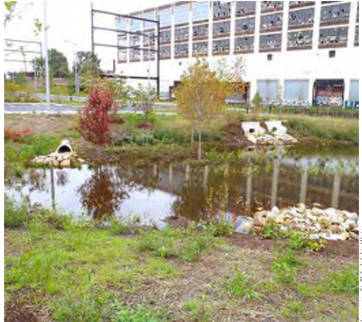
A well-kept stormwater basin.
