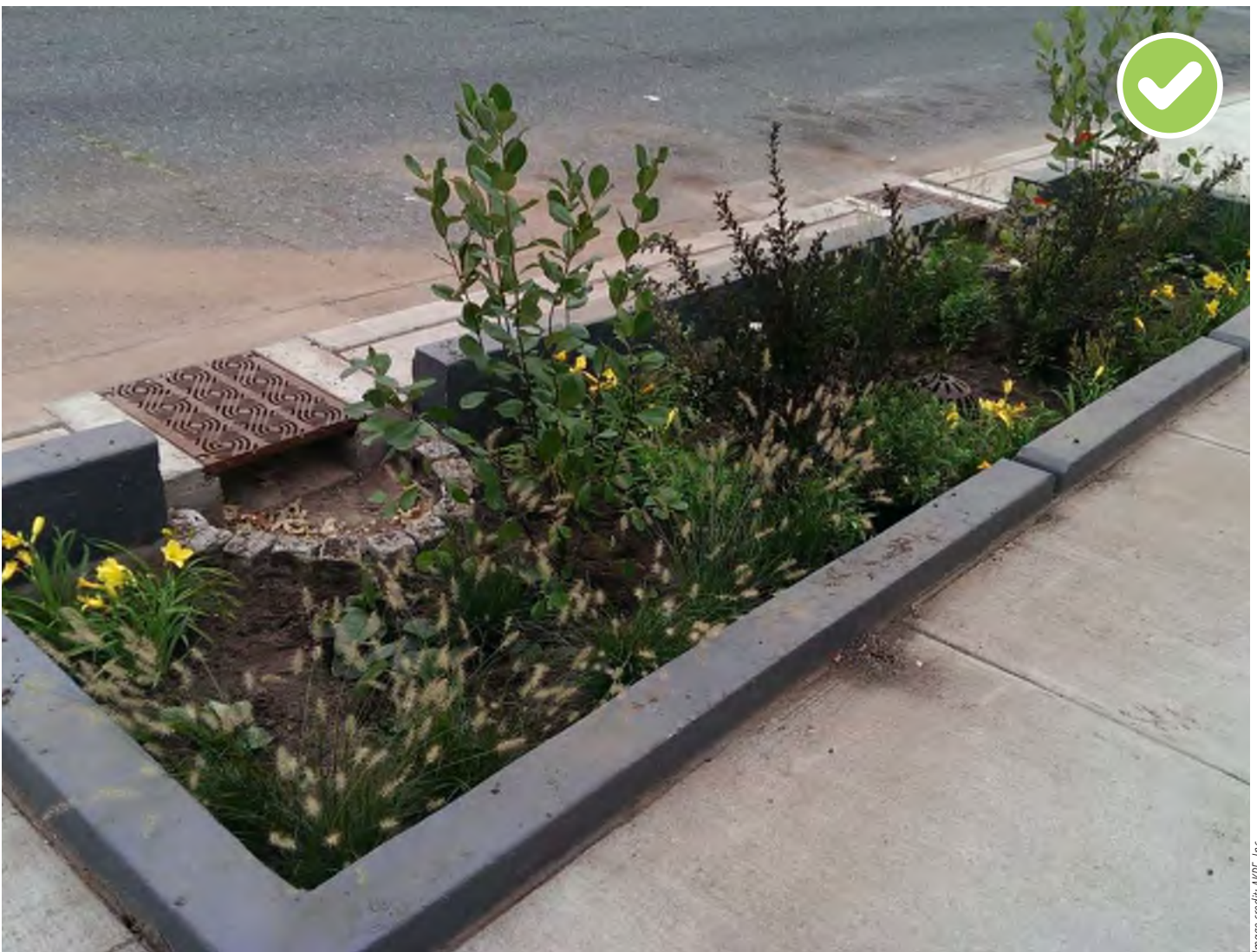
The stormwater planter exemplifies a healthy, well-structured and functioning system.
