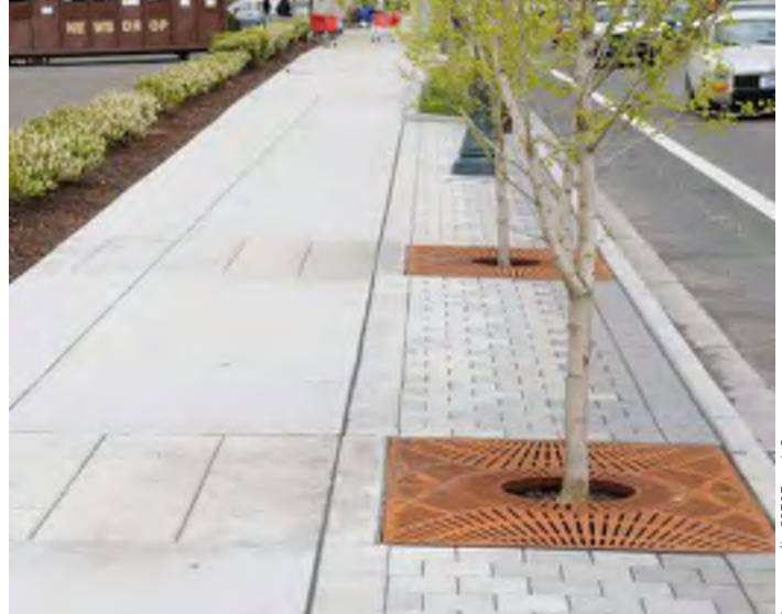
A stormwater tree trench in healthy and clean condition.
