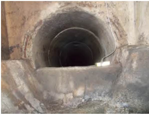
Diversion Weir / CSO Outfall Pipe
