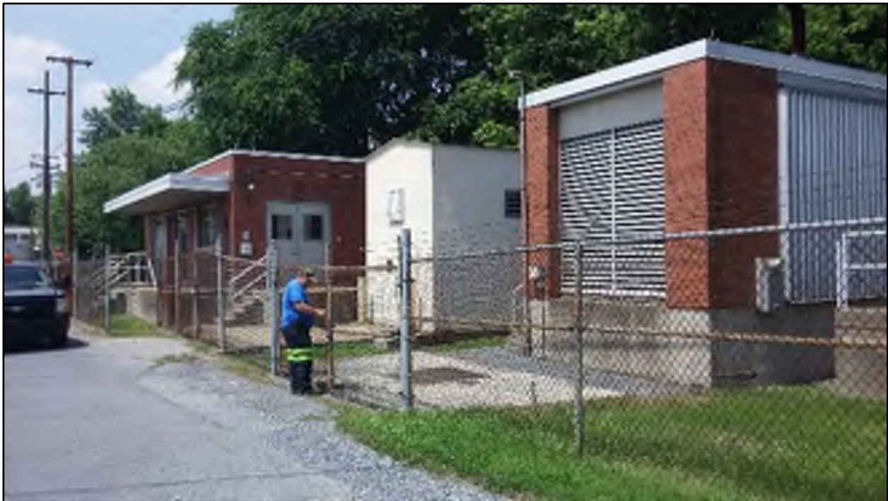
Figure 4.3-7 Spring Creek Pump Station
