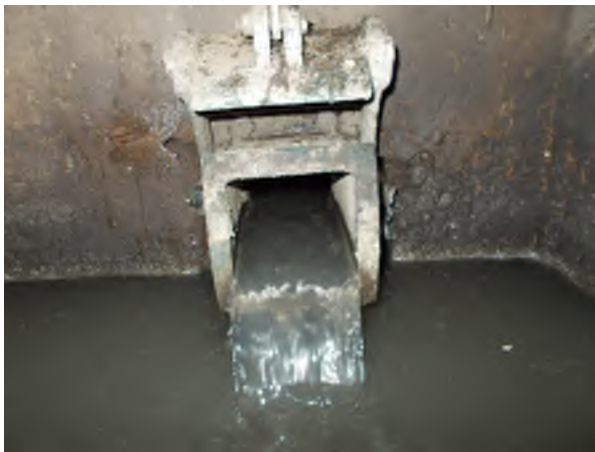
Figure 4.1-4 Photographs of Typical CRW Regulator Structures
