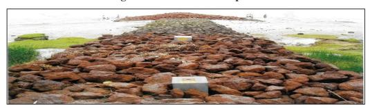
**Image 6.1 Construction of spur**
