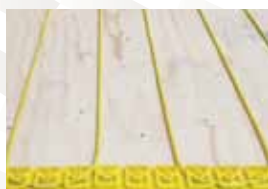
HEATING CABLE INSTALLATION
