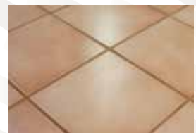
FLOOR COVERING INSTALLATION
