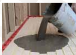
SELF LEVELLING MORTAR APPLICATION
