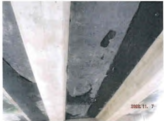
Typical Deck Underside
