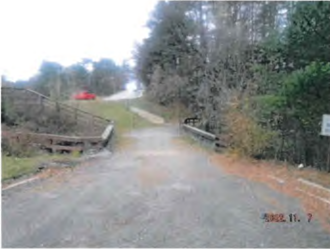
South Approach Looking North
