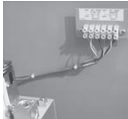
TYPICAL FIELD TERMINATIONS
