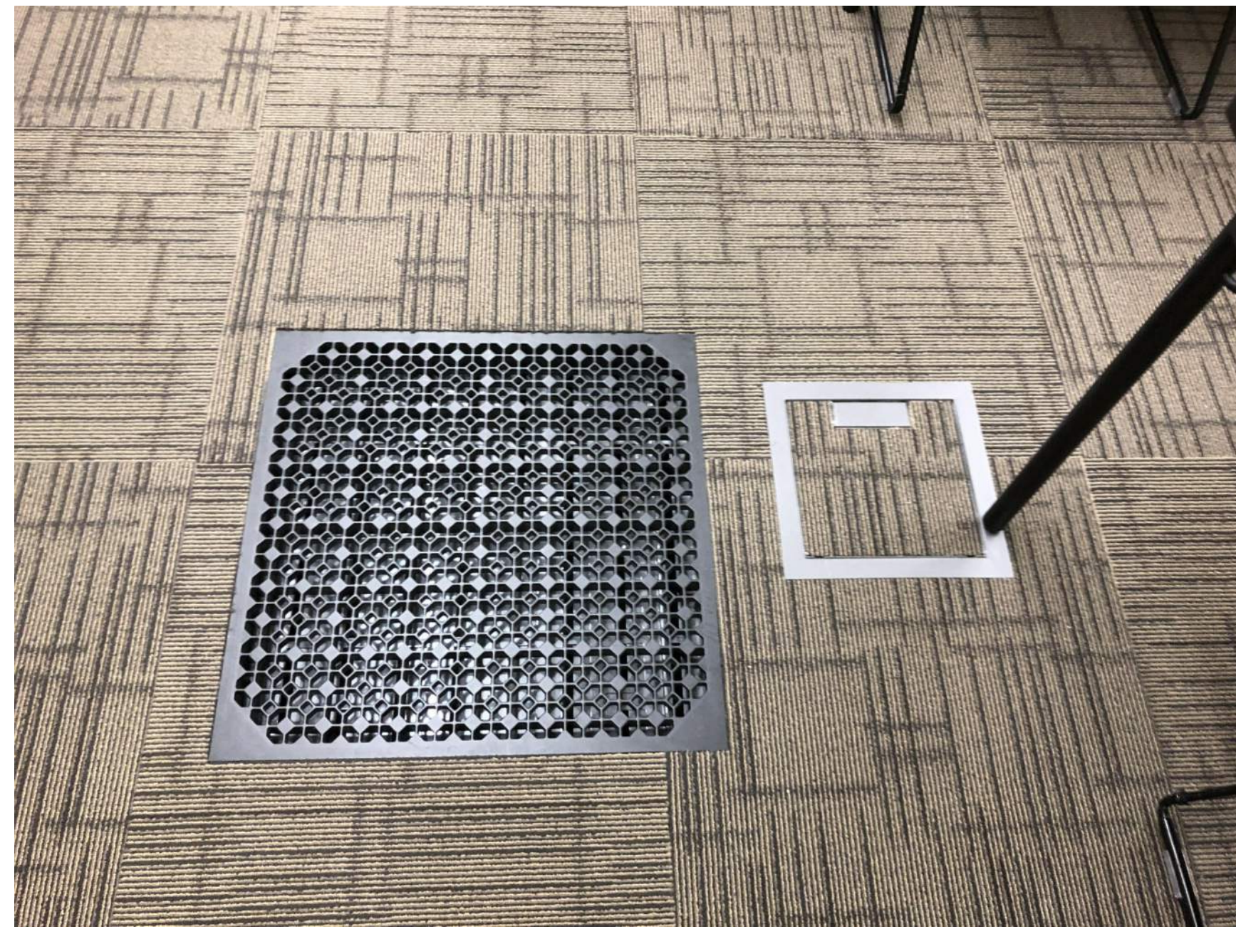
7 EXISTING FLOOR GRATE AND RECEPTACLE 3" = 1'-0"
