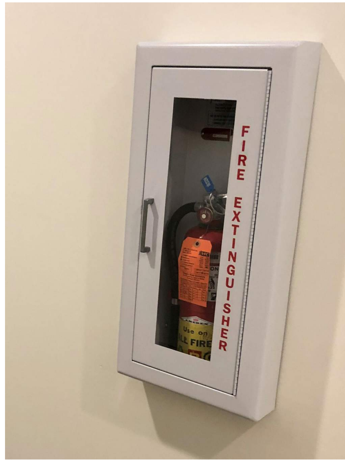
3 EXISTING FIRE EXTINGUISHER CABINET 3" = 1'-0"
