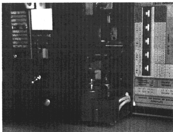
Single Phase Protection and Blown Fuse Indicator
