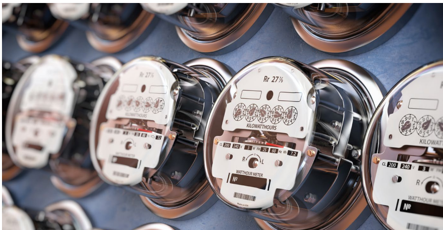
HVAC is the single largest energy consumer in US. ©MSA Safety
