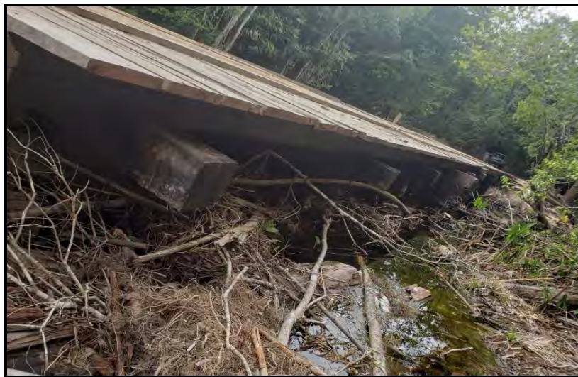
Photographs of the newly rehabilitated timber bridge- 10 July 2023
