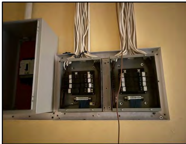
Photographs of the incomplete works - 28 July 2023
