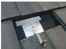
Installed Deck Level Flashing
