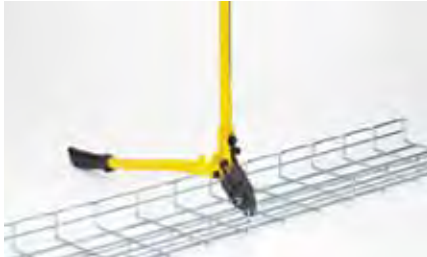
1 Face tray up. Slide cutter next to vertical wire and cut.
