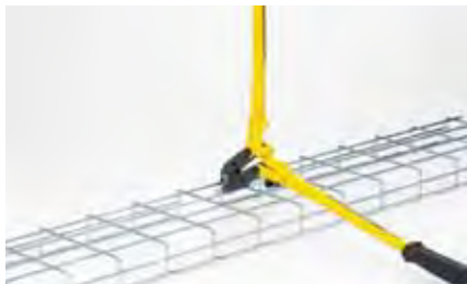
4 Turn tray open-side down and cut wires from bottom of tray.
