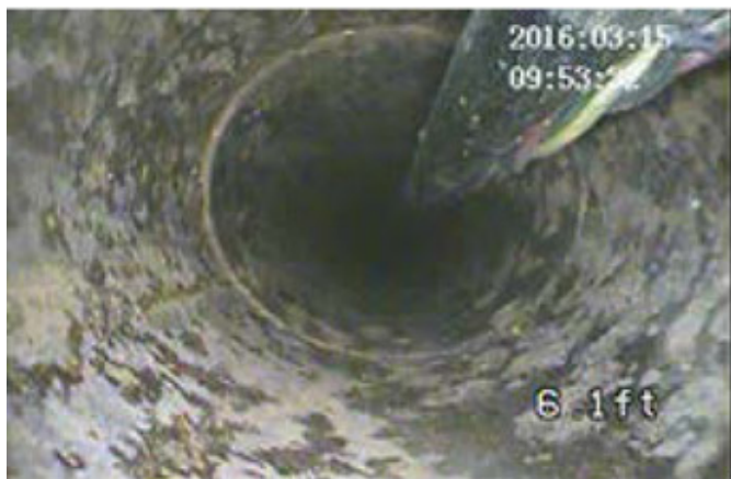
Downhole view of casing joint
