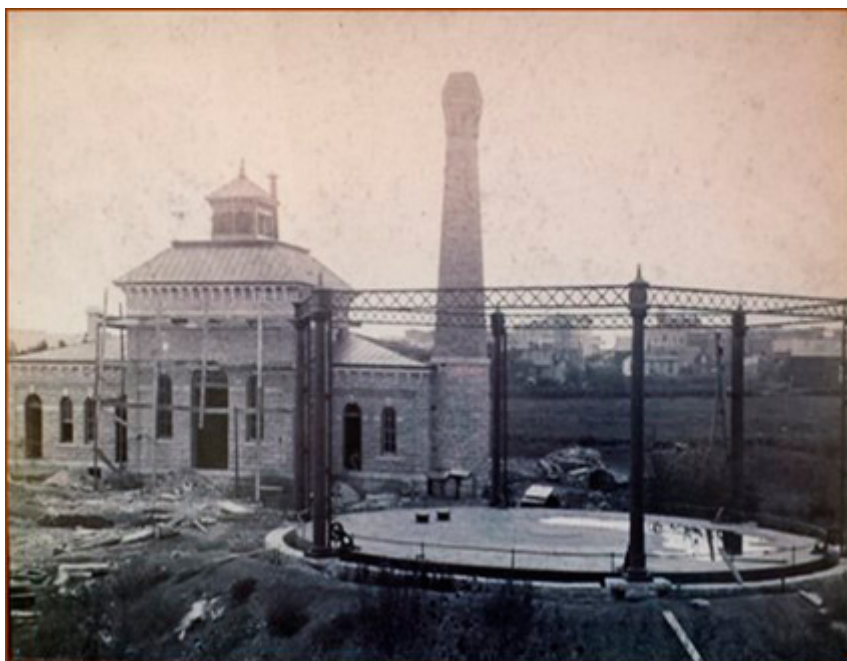
Figure 9-8. Wellington former manufactured gas plant under construction circa 1896. Gas holder in right foreground and plant building at left
