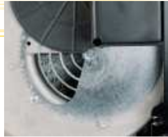
Air damper partially open
