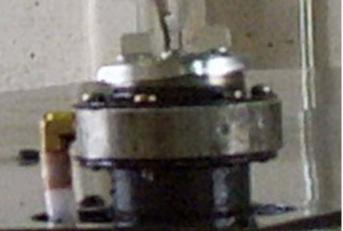
New Spacer For Vent Dryer Installed
