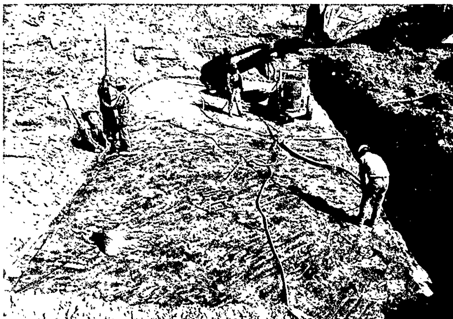
Figure 63. Stilling basin. Spraying aerospray.
