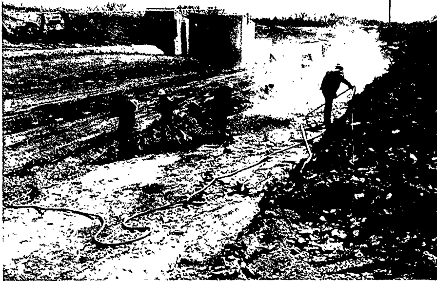
Figure 65. Outlet works, right side looking downstream. Cleaning shale surface in increments prior to placement of fill.
