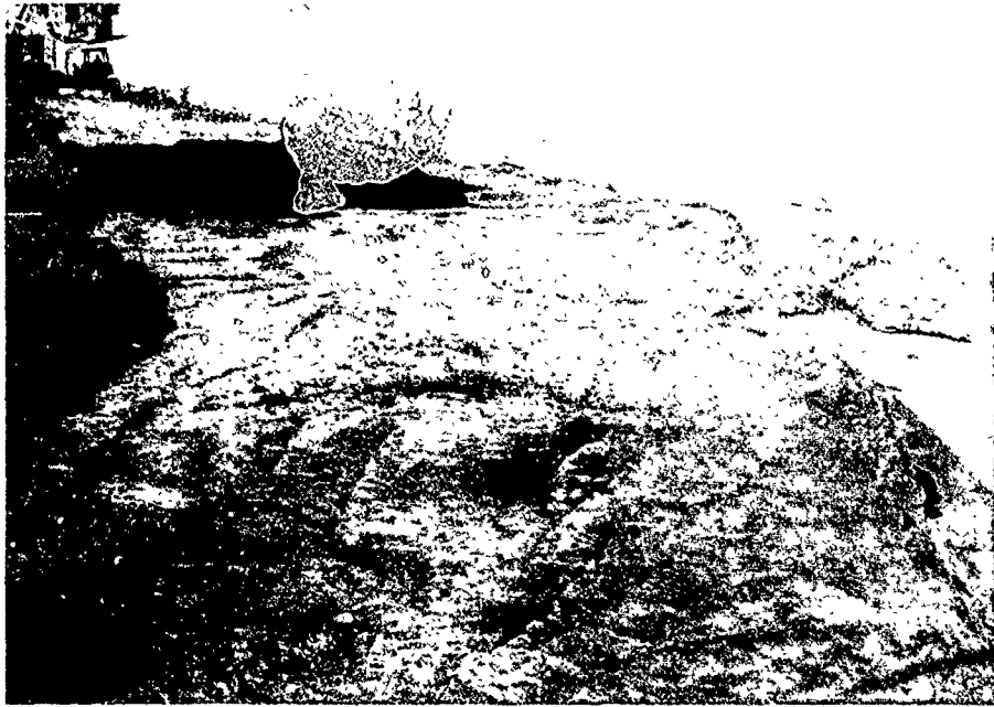
Figure 15. Looking Upstream from valve vault, showing fresh shale surface prior to placement of impervious material.
