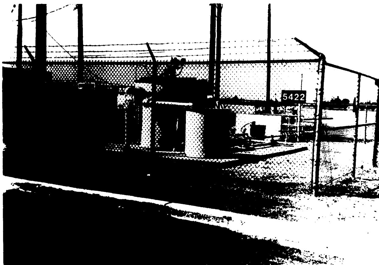
Figure 4. Aircraft Washrack and Separator, Site 40
