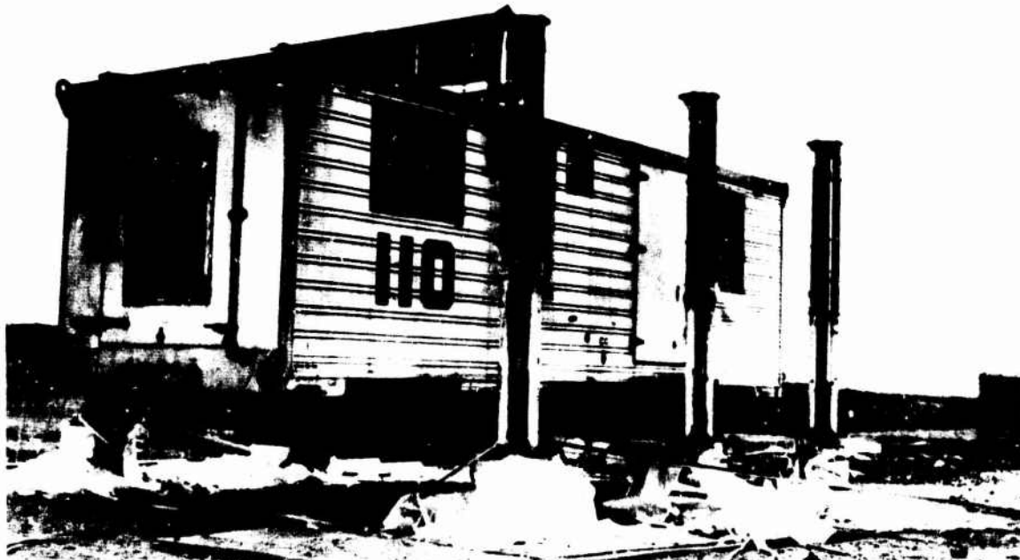
Fig. 13 - Post-shot condition of a typical trailer
