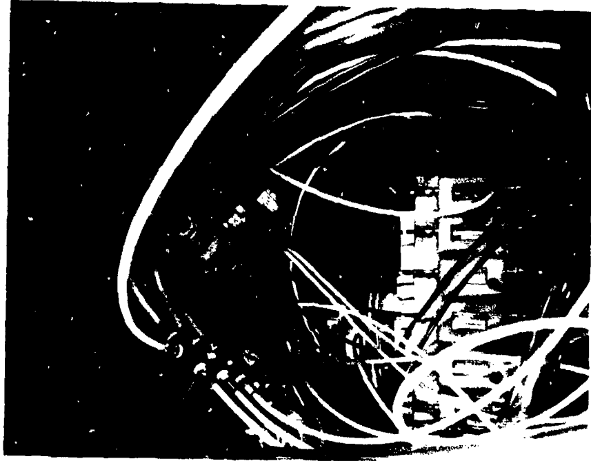
(b) FIBER OPTIC TRANSMITTERS AND SPACE CHARGE DENSITY SAMPLING VALVE ASSEMBLY
