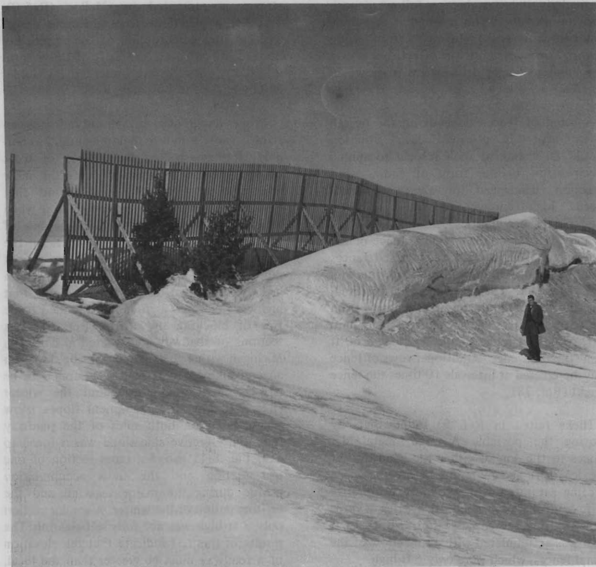
Figure 8-42. Snow Accumulation at a High Snow Fence (12-ft, wood slat drift fence erected permanently along a major highway in Northern Michigan. Note "blow-out" when a section of the fence was removed and not replaced to permit access to cultivated field.) (Photograph supplied by R. W. Gerdel)
