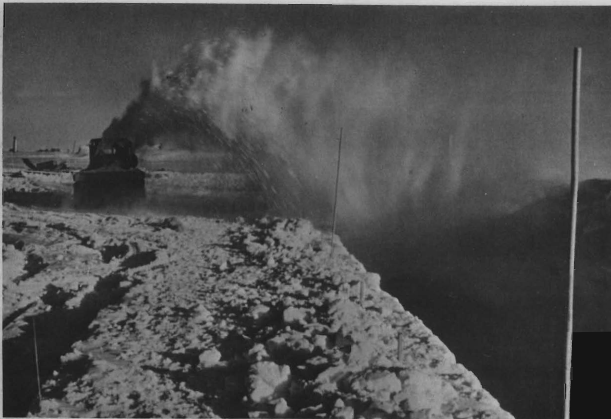
Figure 8-48. Covering Roof Forms at Camp Century, Greenland (Photograph by Waterhouse)
