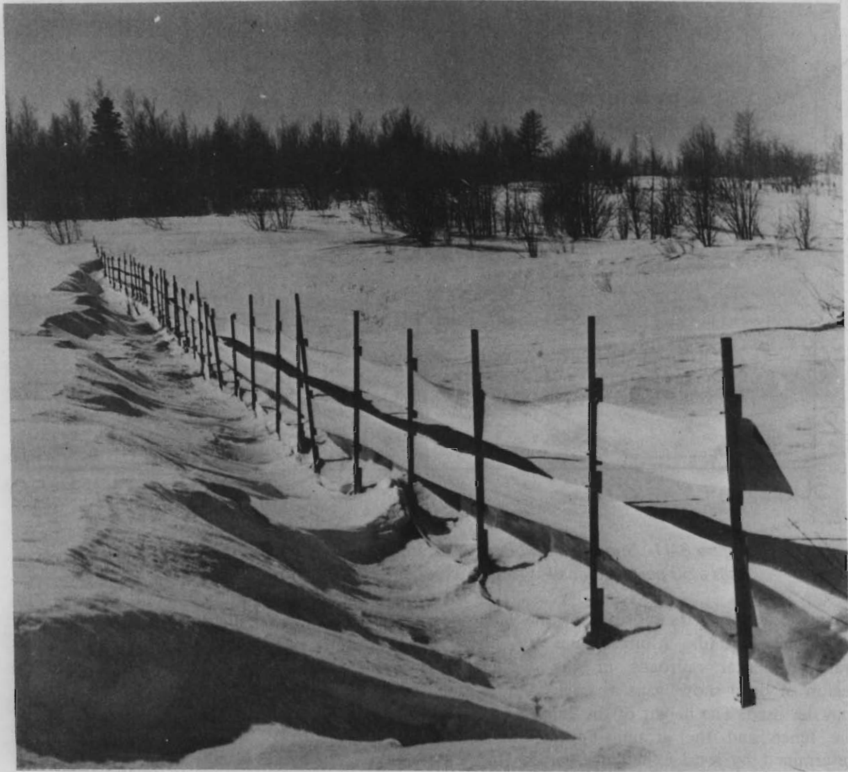
Figure 8-40. Paper Drift Fence (This is shown erected along a highway in Northern Michigan. Note that many more iron fence posts are used than normally required for the common wood slat fence.) (Photograph supplied by R. W. Gerdel)
