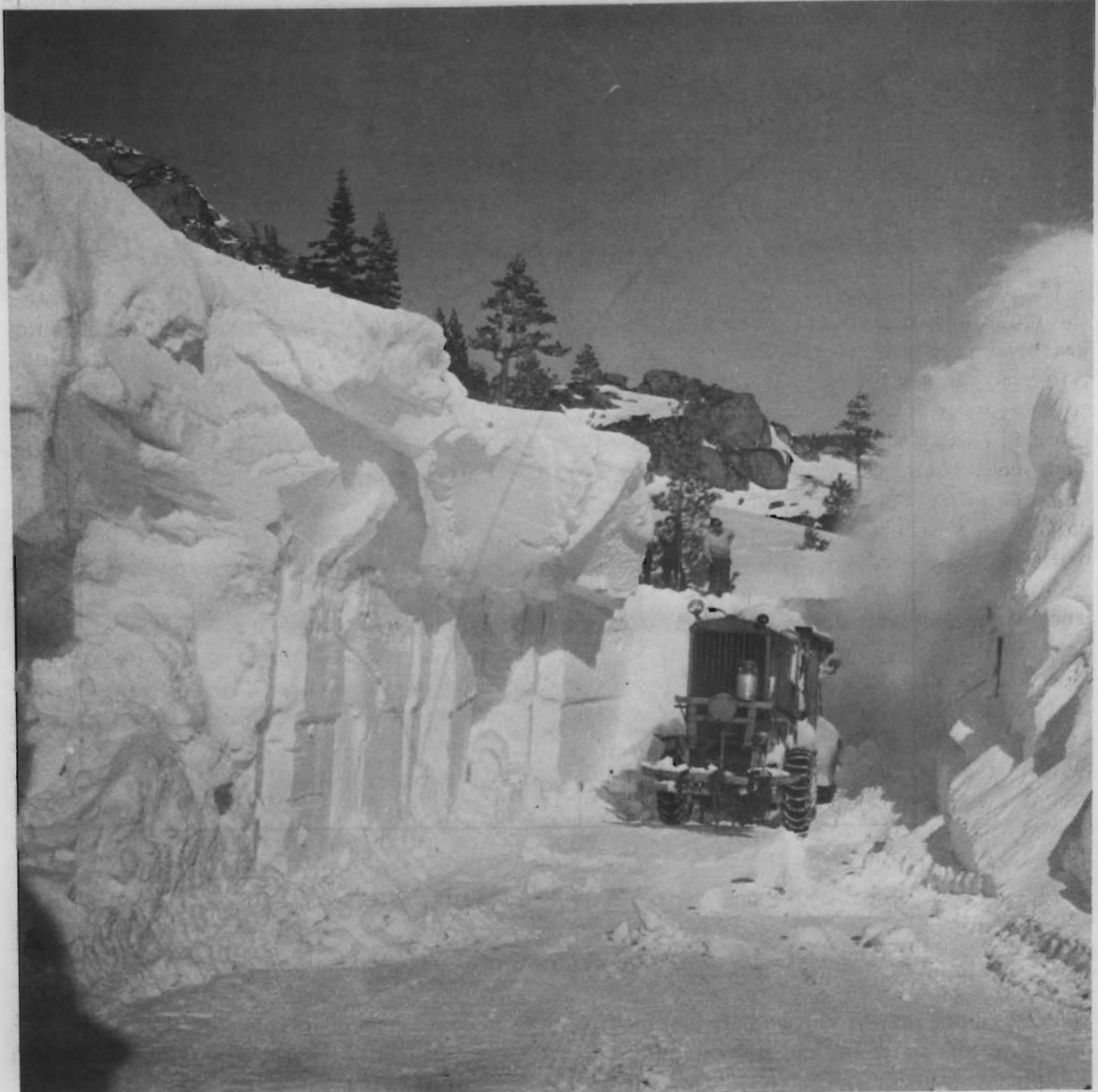
Figure 8-31. Rotary Plow Opening a Mountain Highway (Donner Summit, Calif., following a major snowstorm) (Photograph by R. W. Gerdel)
