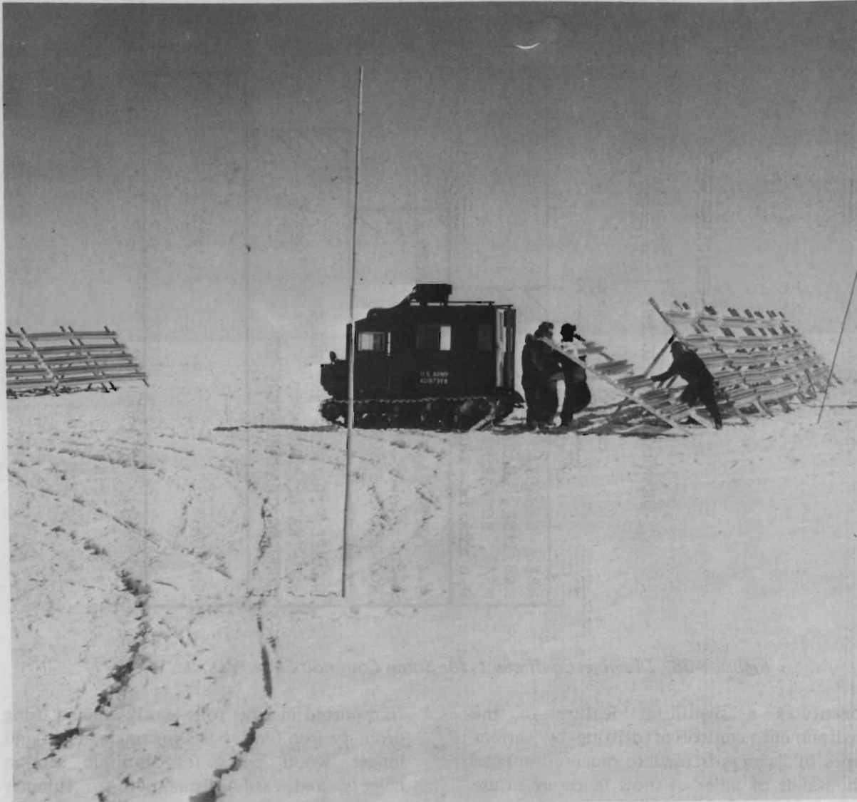
Figure 8-39. All Metal Drift Fences (These are commonly used by railroads and some State Highway Departments. In this photograph the fences are being installed to protect a Greenland Ice Cap facility.) (Photograph by R. W. Gerdel)
