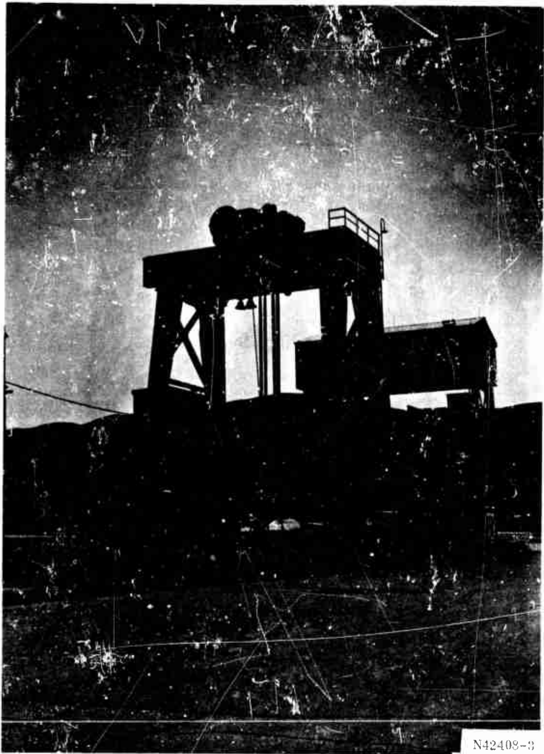
Figure 108. Removing the Loaded Motor from the Casting Pit
