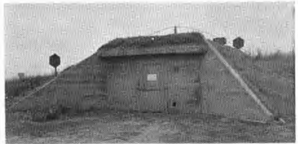
FIGURE 10. Large concrete magazine at Blossom Point.
