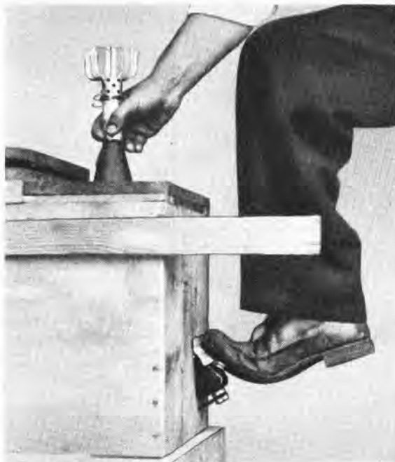
FIGURE 43. Shell being magnetized in magnetization coil.
