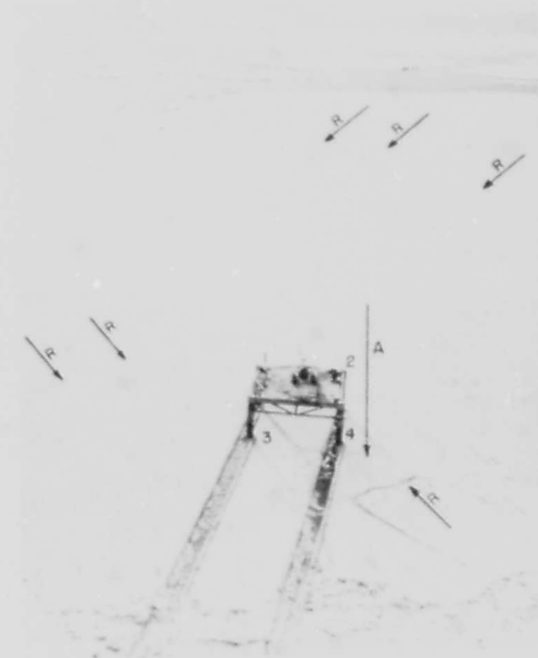
Ice Failure Against Platform II, Note the Double Thick Rafted Section and the Compression Failure on all Four Legs.
