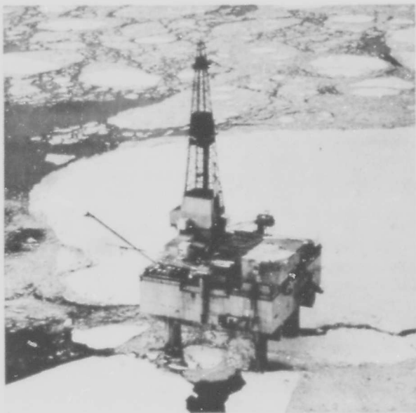
Application of research findings was made in the design of this offshore oil drilling platform in Cook Inlet, Alaska. It has provisions for 32 wells with 8 through each 14.5 foot diameter leg. Eleven such platforms are in various stages of completion.
