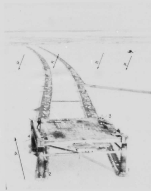
Ice Failure Against Platform, III, Note the Curvilinear Path and Nature of Flow Splitting which does not Reduce Platform Loads.
