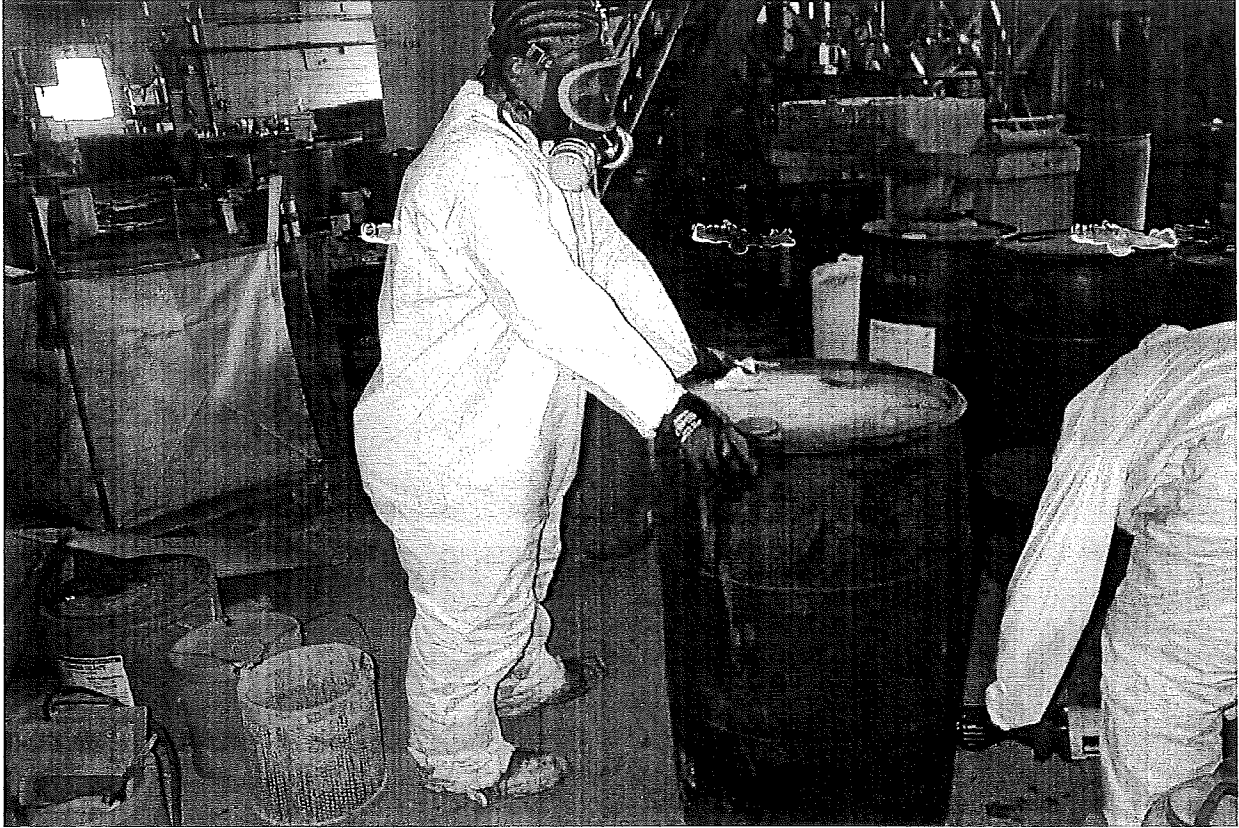
Photo 1: Hazcatting and segregation of drums, vats and containers.
